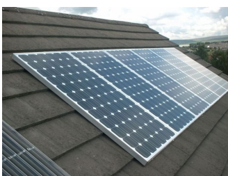
Solar Panels on a Roof
