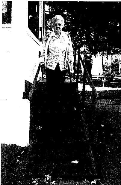
The Elderly Services Agency uses CDBG funds for a small repairs project. A formerly house-bound woman uses her new stairs.
