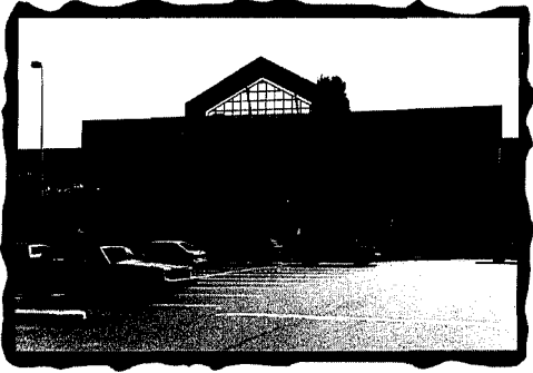
The Promenade Shopping Center, an EDI/Loan Fund project in Seattle, WA.
