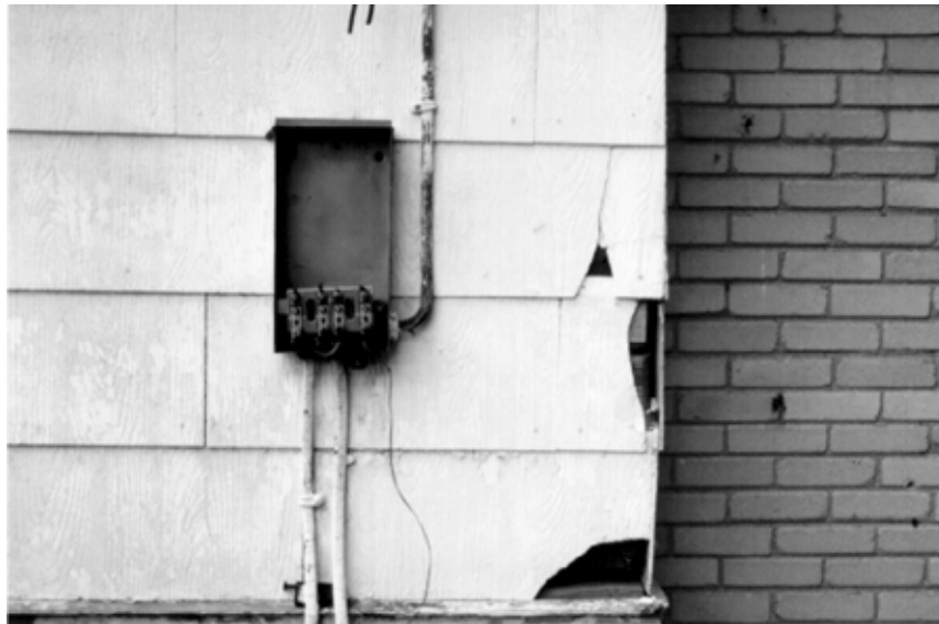
FHA Case Number 261-463489 Detroit, Michigan OIG Inspection May 22, 2000 Exposed Electrical Circuits and Deteriorated Siding
