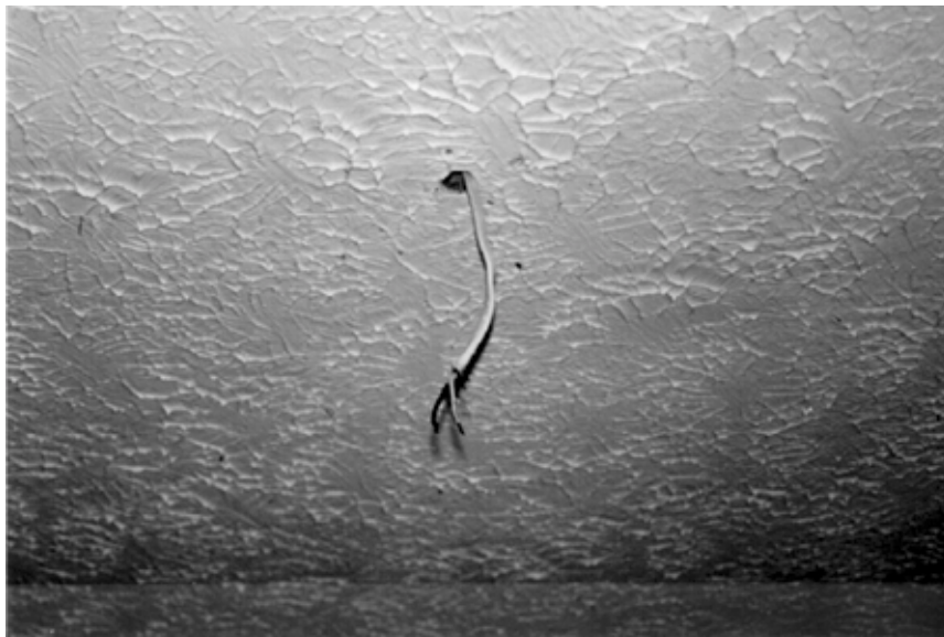
Defective Exterior Paint Surfaces
