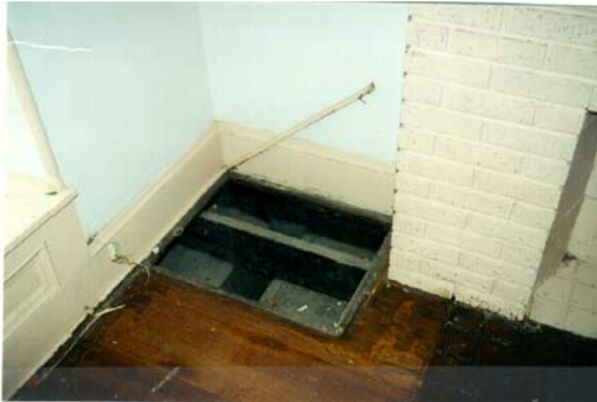
FHA Case Number 412-372302 Cleveland, Ohio OIG Inspection May 31, 2000 Uncovered Hole in Floor
