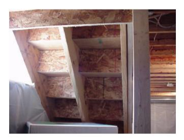
The house at 309 Broadway Street had an undersized floor joist in the laundry room causing the floor to sag in the middle of the room. The floor tiles are cracking as a result of the floor sag.
