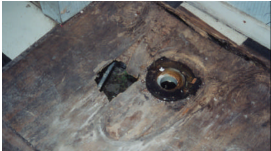
Property case 221-232238, 1638 Clouet St., New Orleans, LA. Toilet has been removed. Sewer gas is allowed to enter unit. The hole in the floor is open to the ground below.
