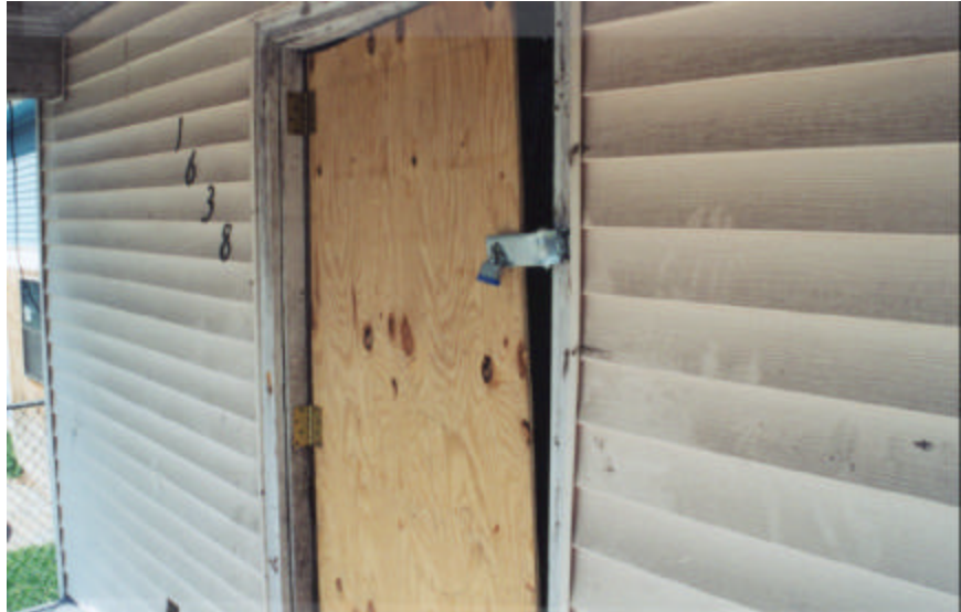
Property case 221-232238, 1638 Clouet St., New Orleans, LA. Front exterior door is missing. Thin sheet of plywood has been substituted. This is not stable or secure. Property is not secured and can be vandalized.
