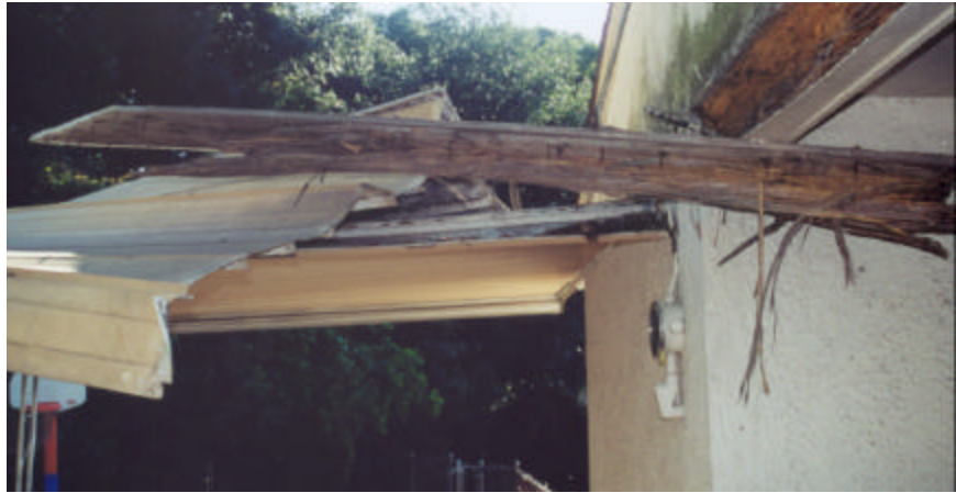
Property case 221-276295, 6945 Downman Rd., New Orleans, LA. Hazardous metal carport roof and termite damaged wood with sharp nails. Requires removal ASAP. The metal roof and/or the damaged wood can fall and cause serious injury.
