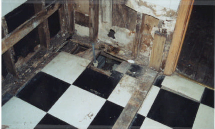
Property case 221-232238, 1638 Clouet St., New Orleans, LA. Bathtub has been removed. The hole in the floor is open to the ground below.
