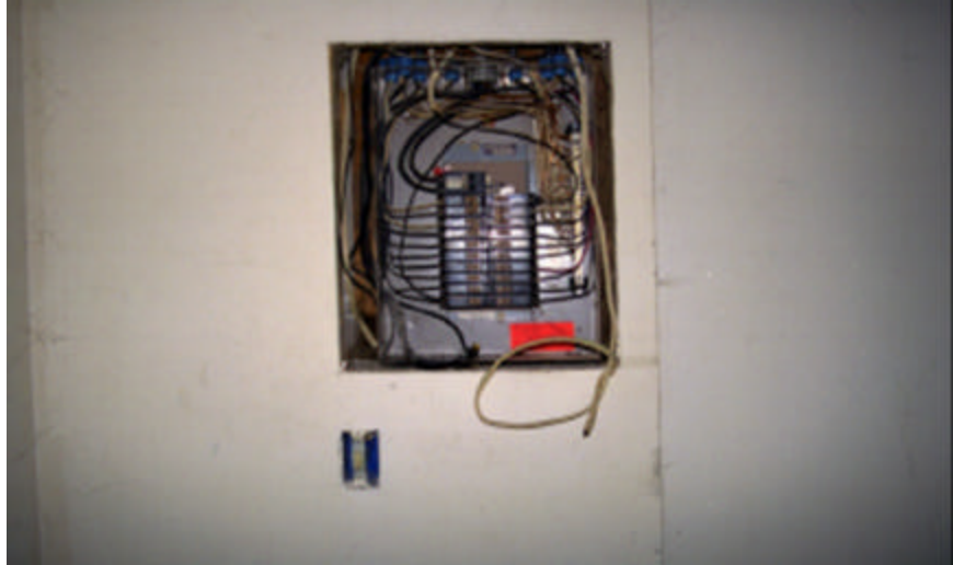
Case 291-188502, 2120 NW 58 th St., Kansas City, MO. Major electrical hazard. Plus missing switch cover plate.
