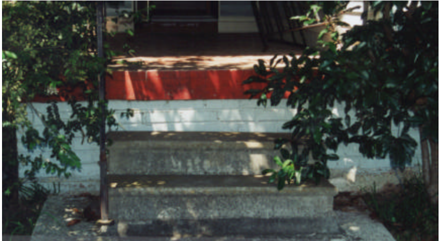
Property case 221-149347, 6400 LaFaye St., New Orleans, LA. Front steps have settled an excessive amount creating a top riser over 8". Very serious tripping hazard.
