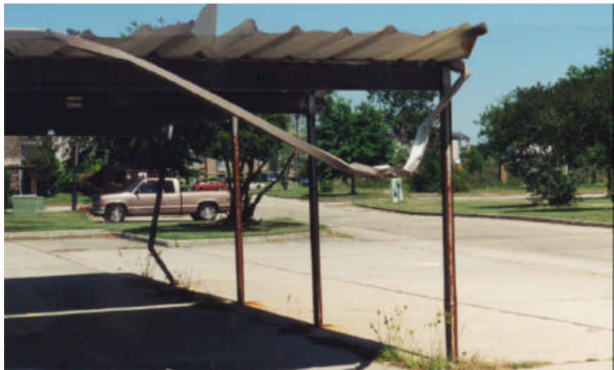
Property case 221-209295, 5505 Bundy, #182, New Orleans, LA. One of several dilapidated and hazardous carport covers in the complex. The cover can fall and cause serious injury.
