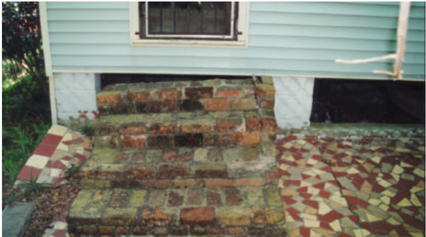
Property case 221-149347, 6400 Lafaye St., New Orleans, LA. Rear steps of the kitchen exterior door has settled excessively. Very hazardous. Proper steps with a 8" riser and a handrail is required.
