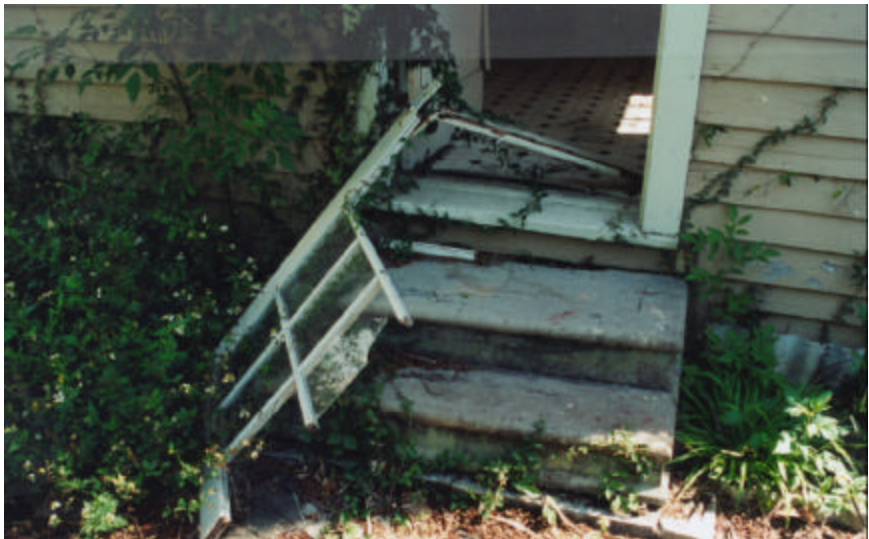
Property case 221-274304, 2720 Onzaga St., New Orleans, LA. Unit has been vandalized by breaking down rear exterior door. The property is exposed to further vandalism and, as evidenced by the growth of vegetation, the door has been broken for an unknown period of time.
