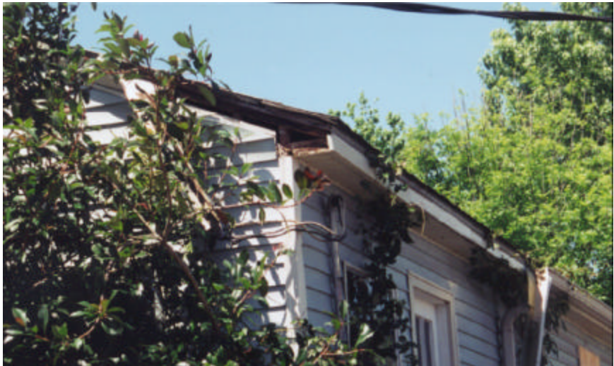
Property case 221-149347, 6400 LaFaye St., New Orleans, LA. Damaged roof fascia at the right front. Also the gutters are damaged. The opening allows excellerated deterioration of the roof and the ceilings.
