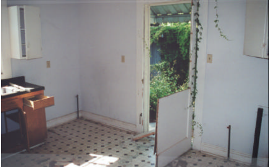
Property case 221-274304, 2720 Onzaga St., New Orleans, LA. Unit has been vandalized by breaking down rear exterior door. The property is exposed to further vandalism and as evidenced by the growth of vegetation on the inside of the property, the door has been broken for an unknown period of time.
