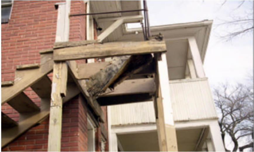
Case 181-980000, 2615 N. 11 th St., Kansas City, KS. Staircase and landing to second floor is rotted away.
