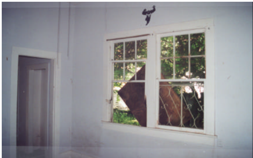
Property case 221-274304, 2720 Onzaga St., New Orleans, LA. Window on the right is missing. Allows entry into the unit. Property is not properly secured and can be vandalized.
