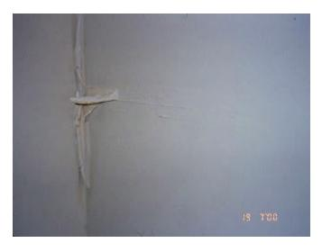
Water is leaking through the wall where the former steam pipes were located in the basement for Building 308.
