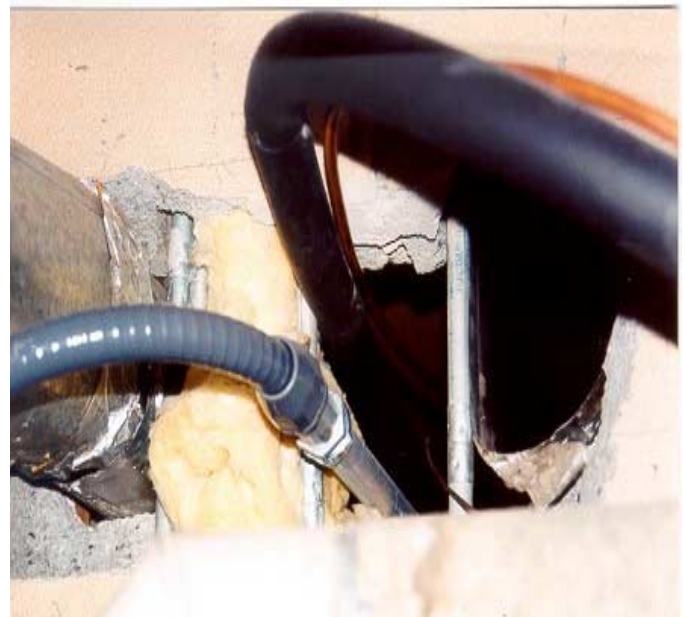
Combustion pipes were not sealed.
