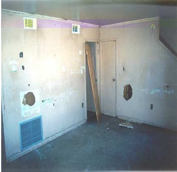
Living room wall was heavily damaged.
