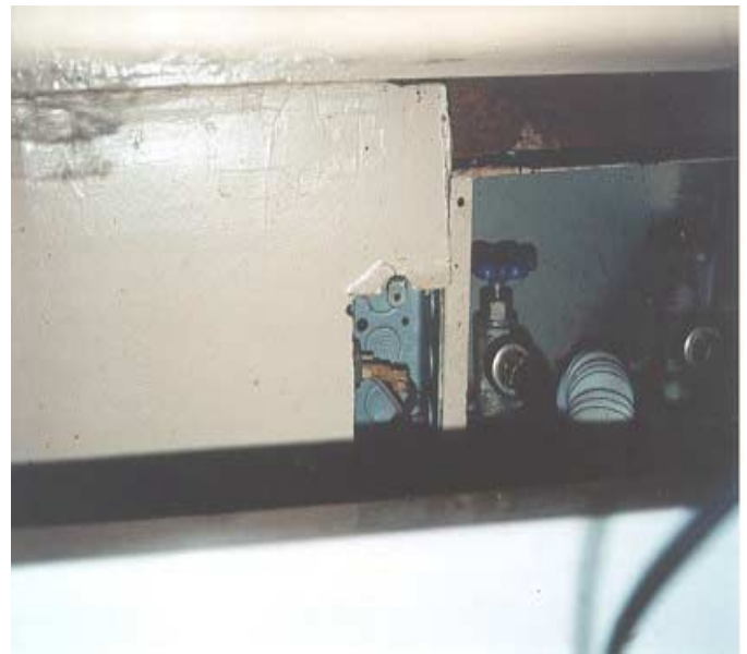
Washer connection for electrical outlet was missing and wiring exposed.
