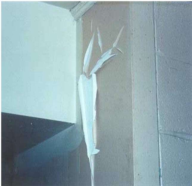
Walls had peeling paint.
