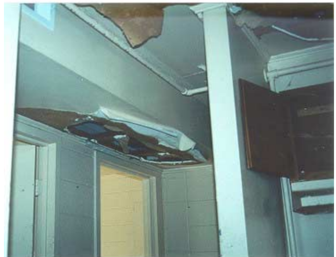
Hall ceiling was damaged.
