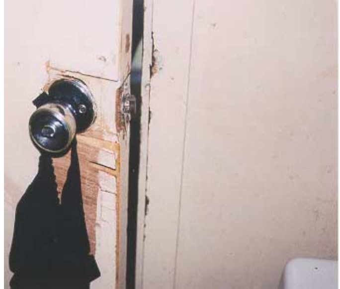
Bathroom door was hazardously damaged.
