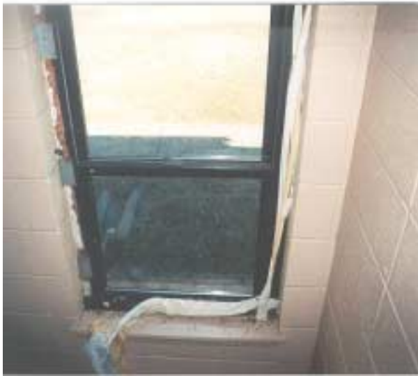
Window was missing perimeter trim.
