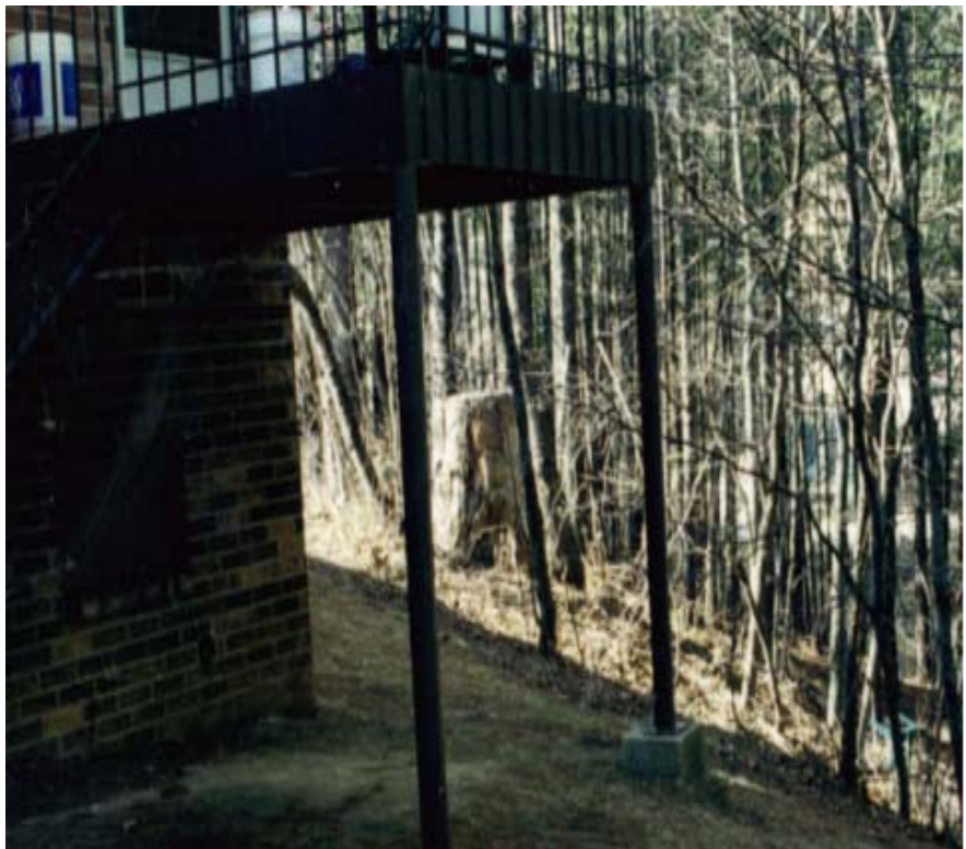
Example of steep, hazardous terrain at Woodland Apartments.
