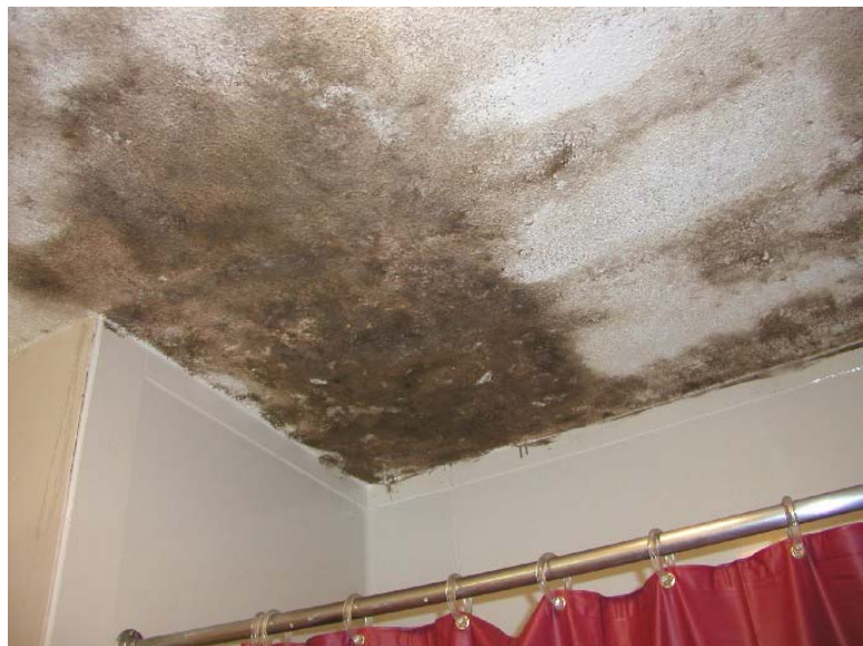
Mold covering Ceiling of Upstairs Bathroom 20 West Clay Street, Unit C
