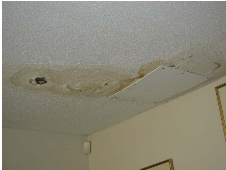
Living room ceiling water stained and damaged 20 West Clay Street, Unit E
