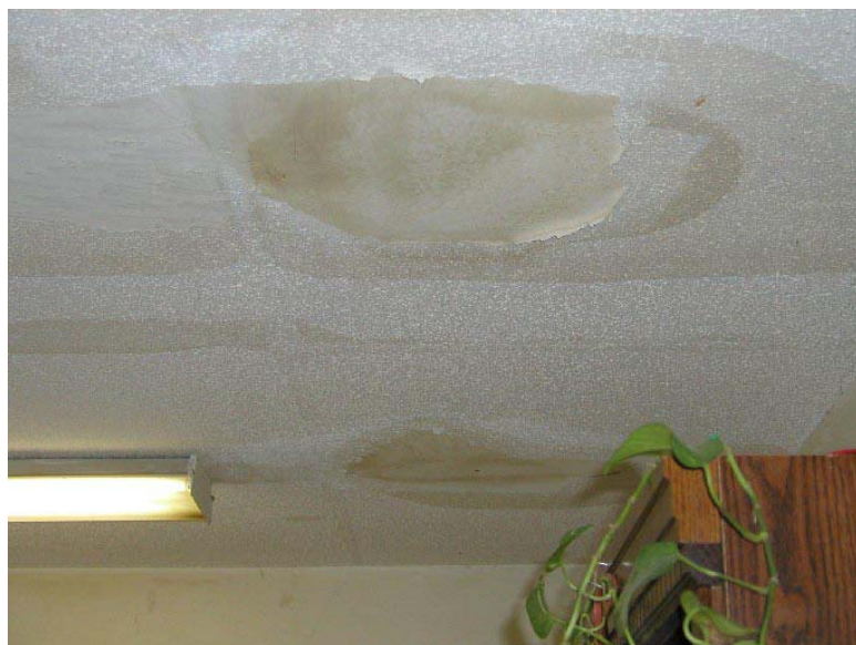
Kitchen Ceiling Water Damaged 10 West Clay Street, Unit C
