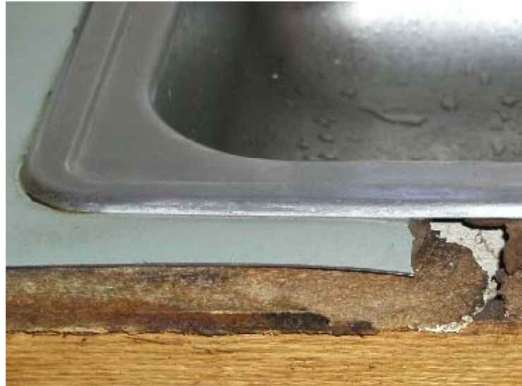
Kitchen Countertop Damaged and Rotted 20 West Clay Street, Unit E
