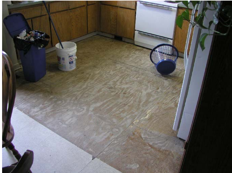
Kitchen Floor Tiles Missing 10 West Clay Street, Unit C
