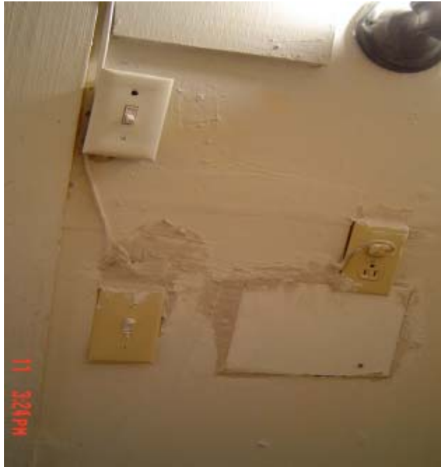
A lamp cord used as permanent wiring
