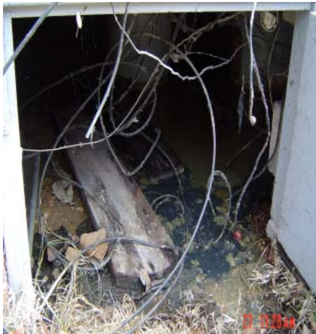
Fecal material from sewage leak under property
