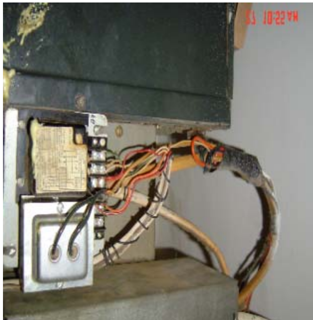
Bare electrical wires at furnace connections
