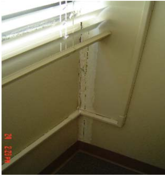
Damage from water leak around window
