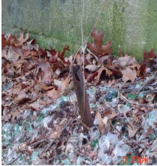
Rusted pipe and broken glass at one unit where two small children lived
