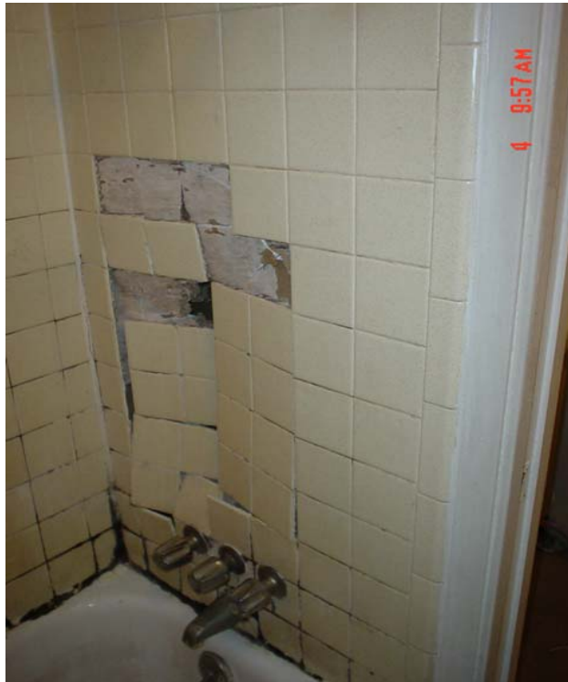
Wall damage and buckled tiles in a unit's bathroom.
