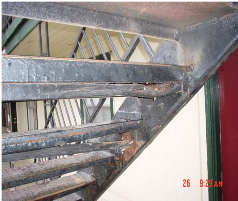
Unsafe stairs to a unit, which contained risers that were rotted and rusted free from the supports.
