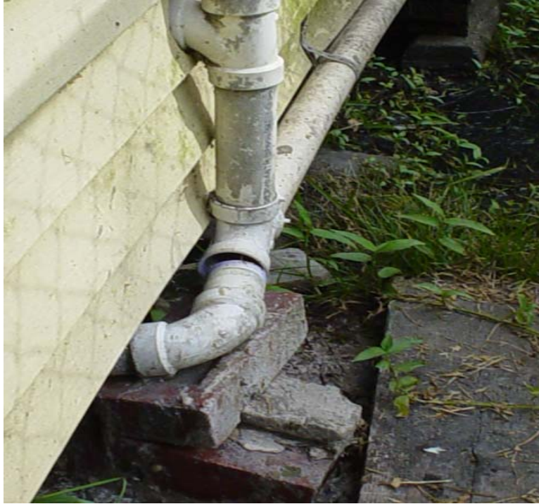
Improperly supported main sewer drain line leaking under the house. Sewage had been leaking out so long it was pooling under the house, in the backyard and affecting the house's foundation.
