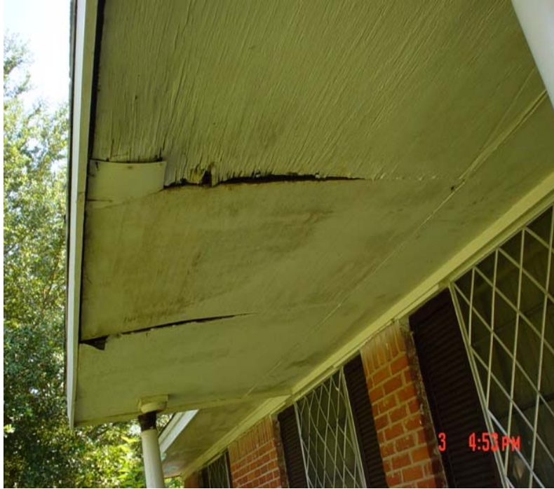
Water damaged and rotted porch ceiling. Further, the support column, shown in the lower left, has slipped forward and is not properly supporting the weight of the porch.
