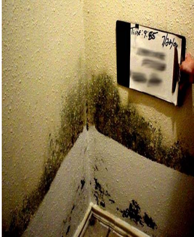
Bedroom has mold growing above and through new paint because the owner did not correct the underlying moisture cause.
