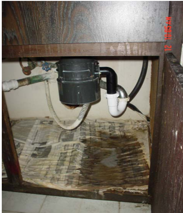
Leaking garbage disposal and rotted cabinet.
