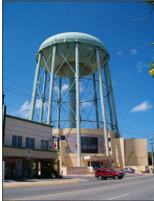
Picture of the front of the public library. The library is beneath the water tower and has no parking facility.
