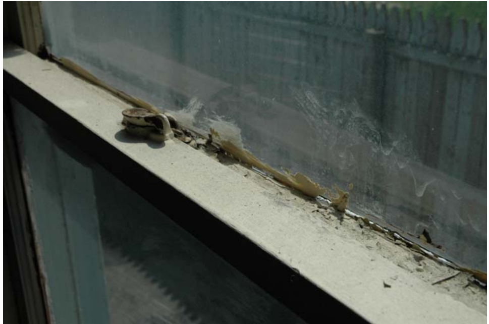
Unit #1000093: Right rear bedroom window does not align to lock.
