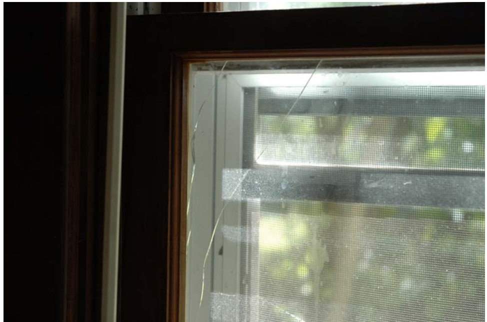
Unit #1000080: Cracked glass pane on kitchen window.
