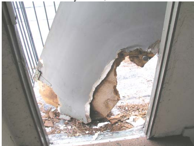
Damaged roof access door
