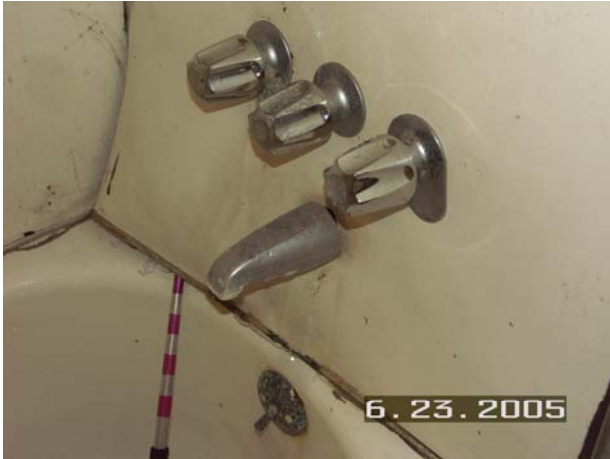
Tub wall separating and deteriorating
