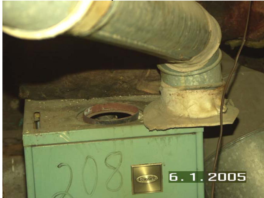
Furnace exhaust not ventilating to exterior of building.
