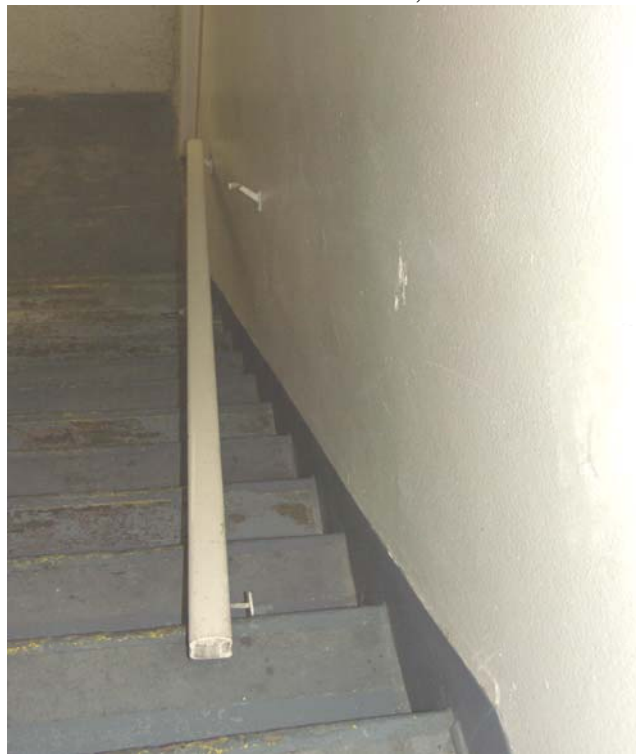
Detached handrail in common area
