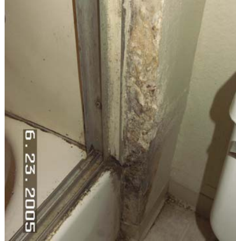
Tub wall separating and deteriorating
