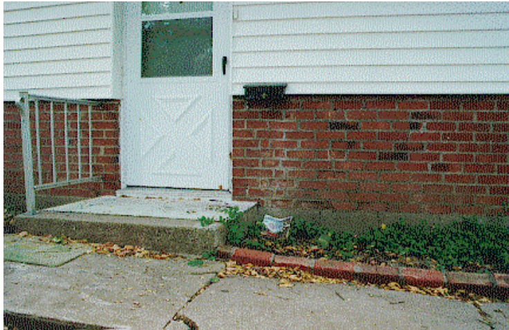
Figure 1: 6733 Bellefontaine-Bricks are crumbling away from house around entry.
