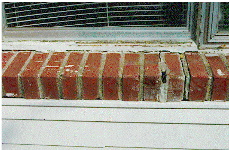
Figure 2: 6733 Bellefontaine-Bricks are crumbling away from house around windows.
