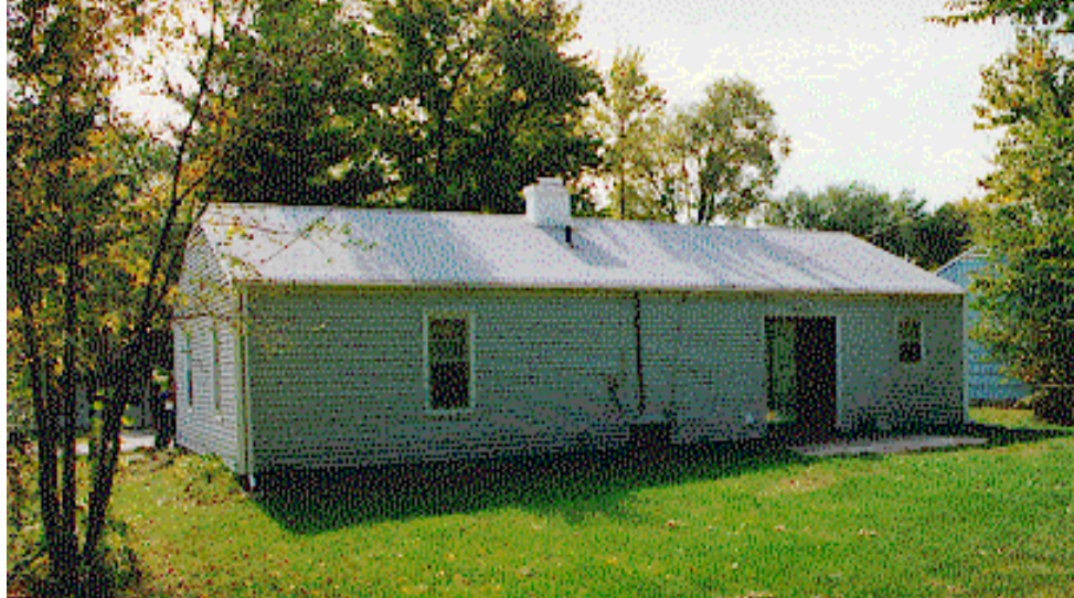
Figure 3: 8406 East 111th Street-House has no masonry or stairs in front.
