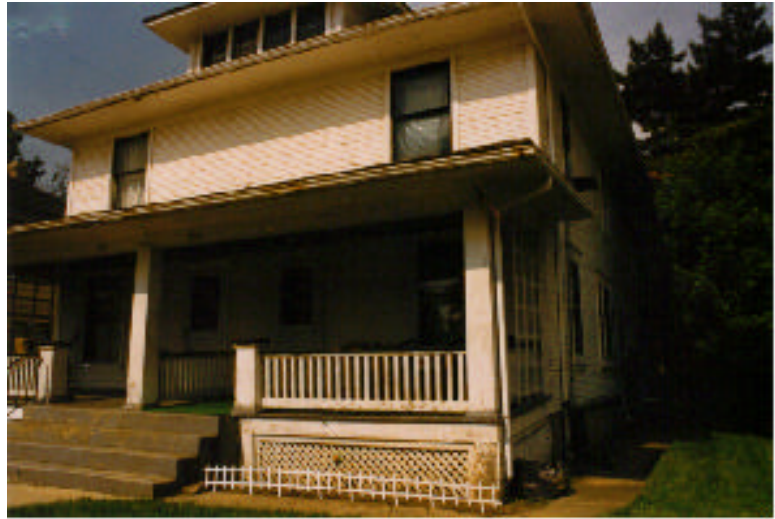
No handrail for front porch steps at 1311 Clifton
