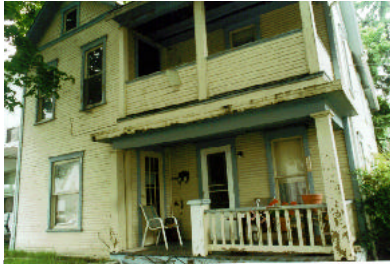
Peeling paint on exterior siding and front porch at 1834 Highland
