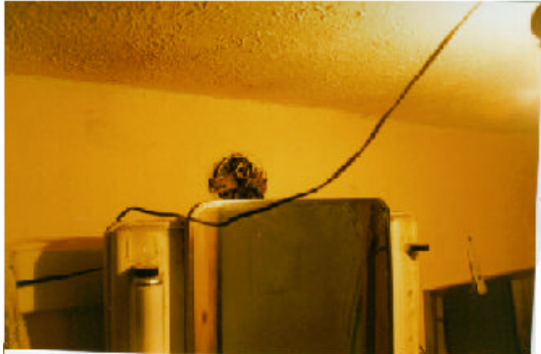
Improper wiring and exposed wiring for light fixture in bathroom above sink at 1554 Sheridan, Apt. 2
