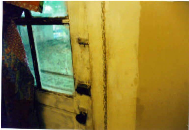
The back door was missing the half of the locking mechanism on the door frame at 1834 Highland
