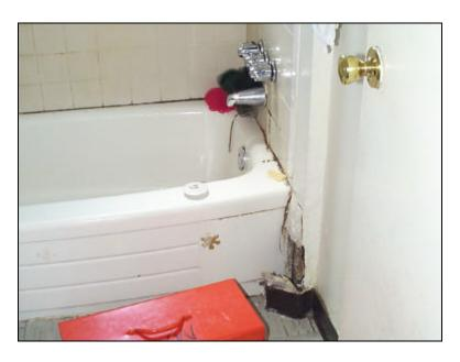
The apartment at 9110 Hough Avenue for Park Village had missing ceramic tile and drywall. The resident taped plastic over the hole to avoid further damage.
