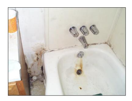
The apartment at 2521 East 33<sup>rd</sup> Street for Longwood had damaged drywall and the bathtub caulking needed to be replaced.
