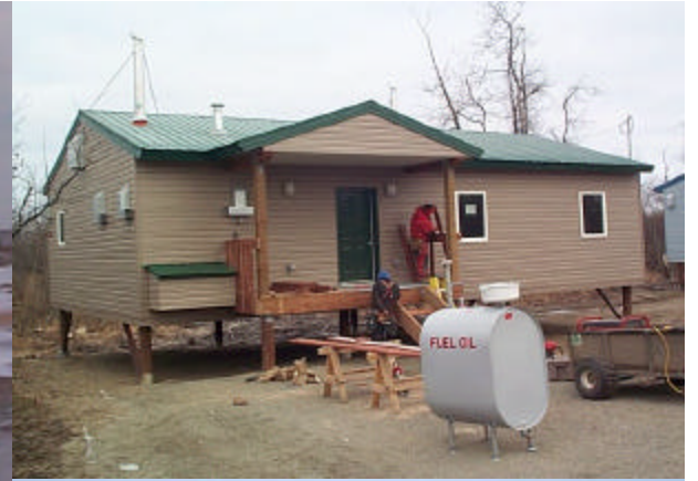
AVCP 220 UNIT #3 IN PROCESS OF BEING LOWERED ONTO THE PILE FOUNDATION. (3-13-01)
