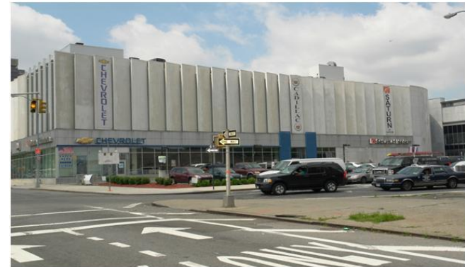
Harlem Auto Mall After Completion
