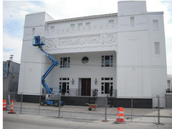
During Recent Renovations
