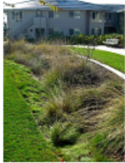
BIOSWALE WITH 3:1 SLOPE ON BOTH SIDES AND 3' OFFSET FROM THE PARKING LOTS ON EITHER SIDES
