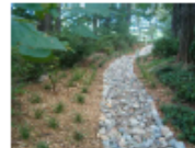
OVERFLOW SWALE WITH CHANNEL PROTECTION AND STONE WALL REINFORCEMENT OUTFILL BALANCE AREA
