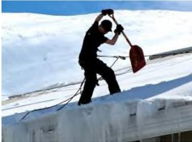
Employees might need to climb directly onto the roof and use equipment such as shovels, snow rakes, snow blowers and ladders. These operations may also be performed from the ground level using snow rakes. Aerial lifts are sometimes used to access roofs and apply de-icing materials. Snow, ice, and wind can make it difficult for contractors to maintain their footing and grip while working in the winter.
