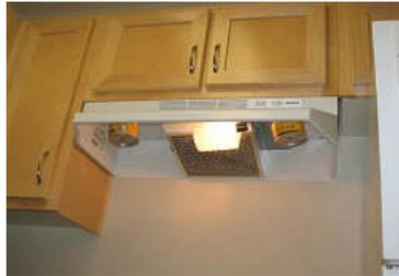
the flame reaches the canisters, the fire suppressing powder is automatically released onto the fire. After the stove has been turned off and is cool to the touch, the powder can be cleaned-up with a vacuum and wet cloth.
