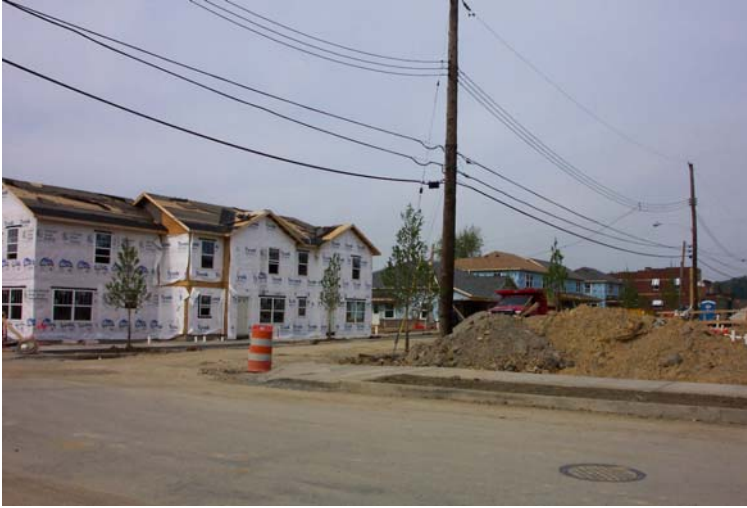
Scattered site duplexes and triplexes under construction in Clairton, PA
