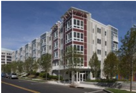
Above: Newly completed Metro Green residences in Stamford, CT.
