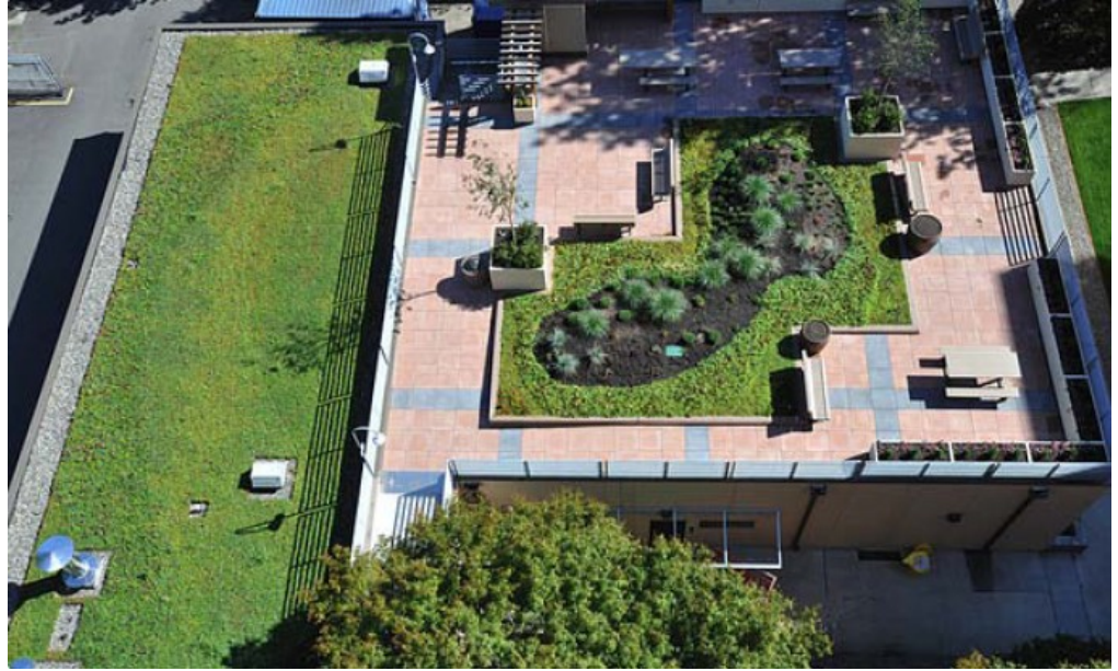
Completed green roof at Lincoln Square
