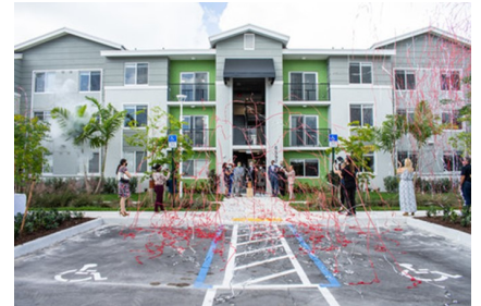
Liberty Square Phase II consists of 204 units; 73 are public housing apartments
