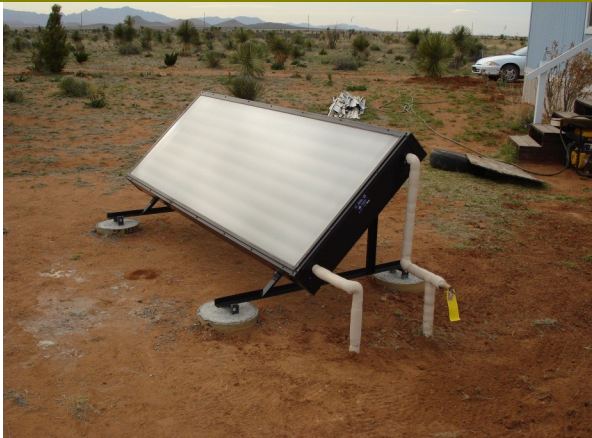
Typical Residential Solar Hot water installation
