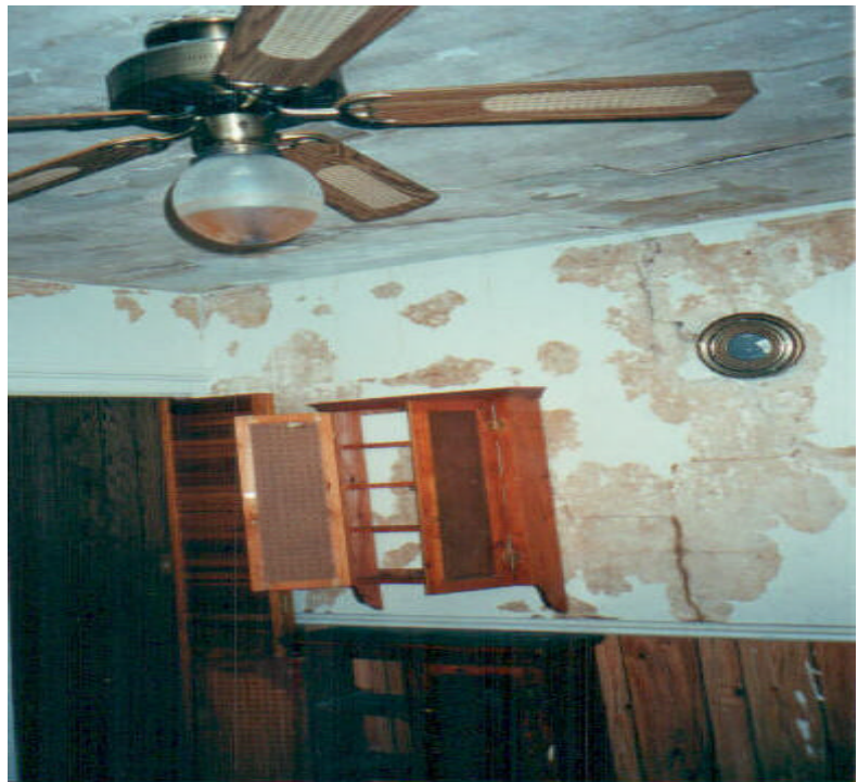
FHA Case No. 061-070356 - Defective paint, water in light fixture
