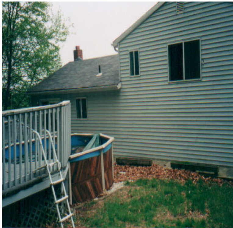
FHA Case No. 061-152960 - Improperly covered pool
