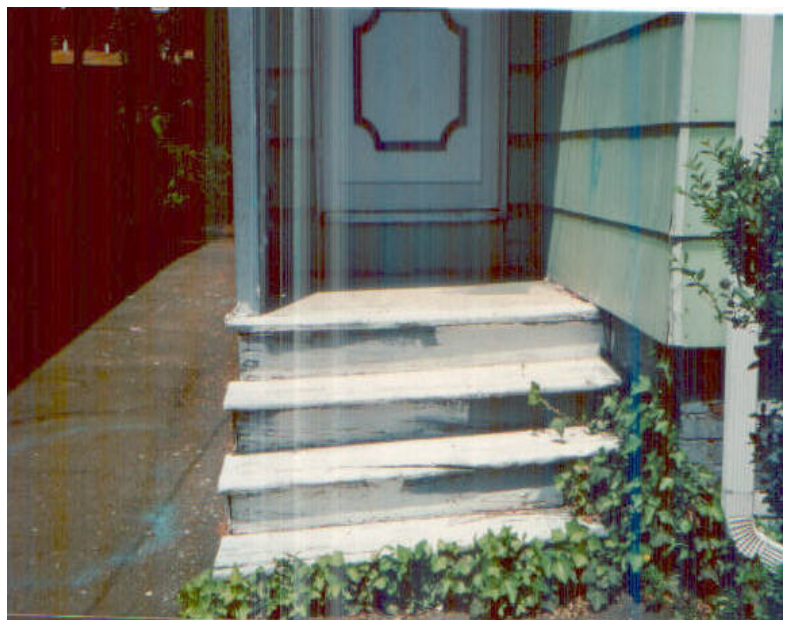
FHA Case No. 061-068871 - Decayed front Step
