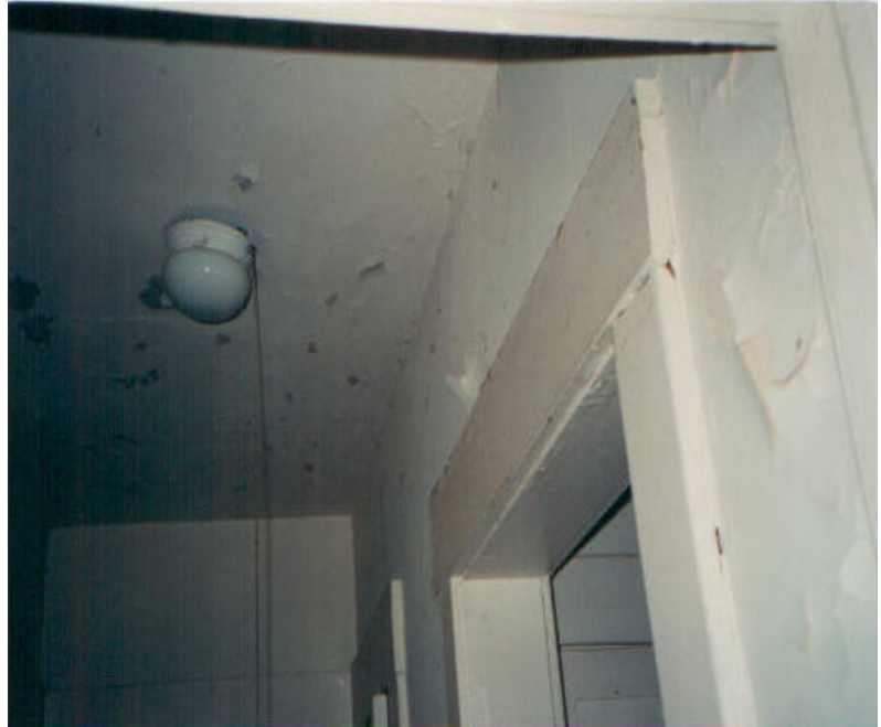
FHA Case No. 061-071714 - Defective paint
