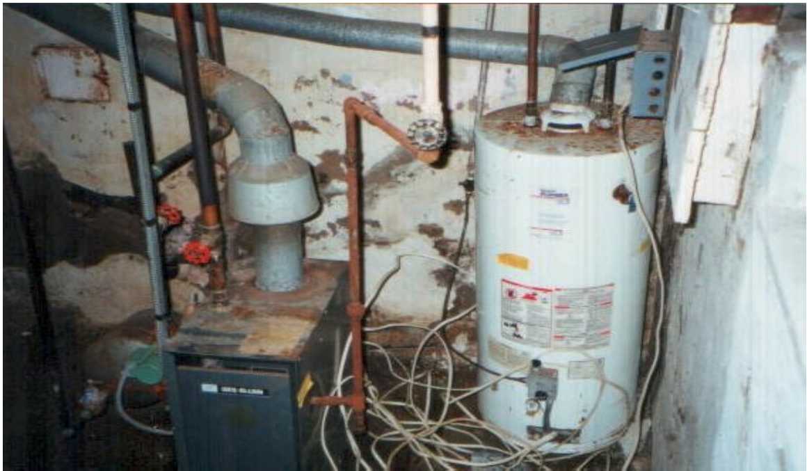
Acquired: 08-13-99 Case No: 372-265070 OIG Inspection: 06-01-00 Location: Buffalo, NY Condition: Mass of wiring is an electrical hazard.
