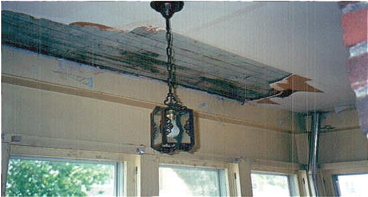
Acquired: 12-11-99 Case No: 441-444362 OIG Inspection: 06-08-00 Location: Philadelphia, PA Condition: Roof leaks have caused significant ceiling damage
