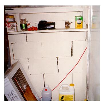
The house at 2001 Livingston Avenue, Wellston had a crack in the foundation that was not addressed during the housing rehabilitation work. The amount of needed repairs for this house exceeded the State's maximum assistance allowance. The house at 2135 Carroll-Eastern Road, Pleasantville was missing an electrical outlet cover plate, the outlet was not secured to the wall, and the wiring was not replaced as required by the housing rehabilitation contract.
