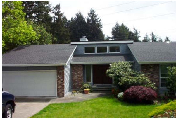
Exterior of home 2
