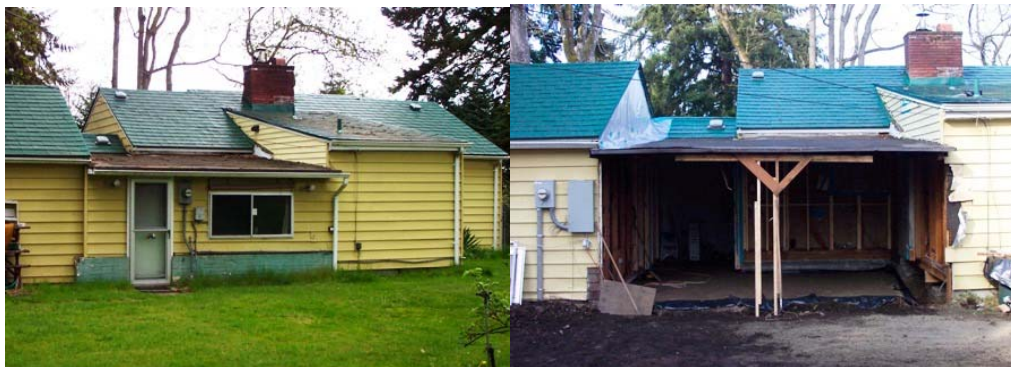
Enclosed porch before and during demolition
