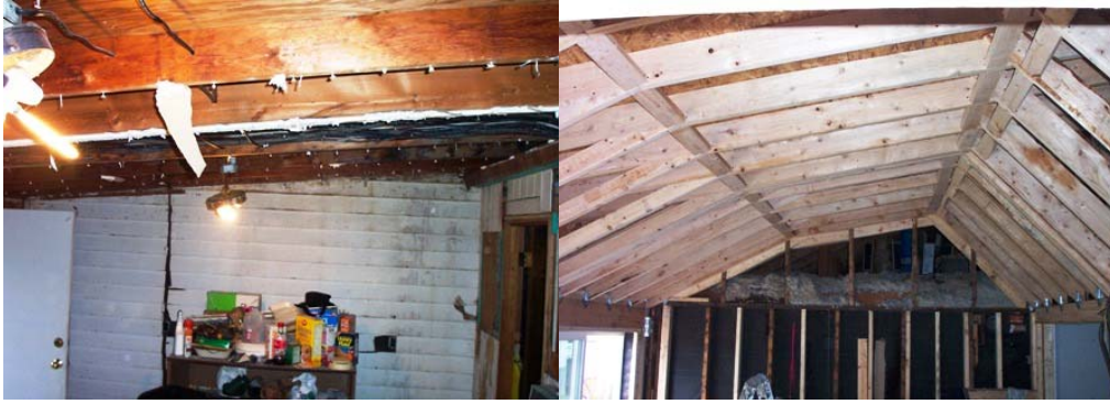
Inside before demolition and during reconstruction
