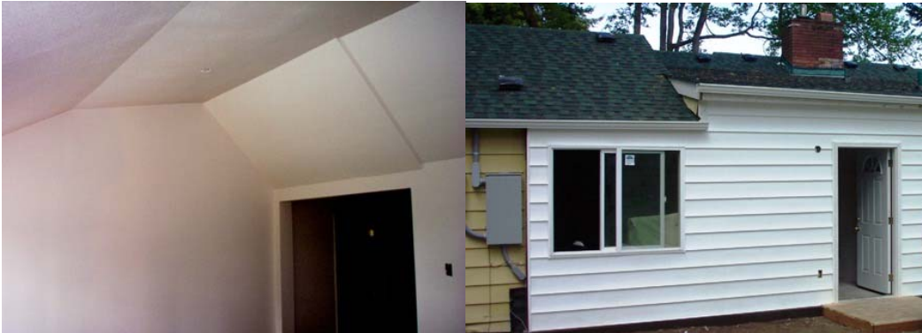
Inside and outside finished (before painting)
