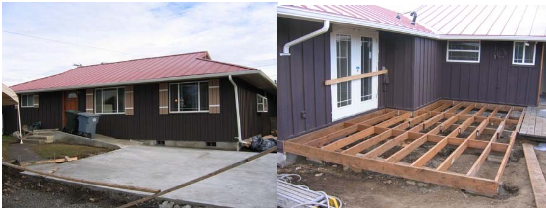
After rehabilitation (Deck was not paid for with HOME funds.)
