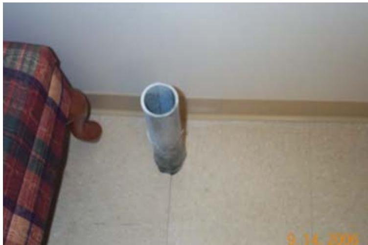
Pipe from first floor water closet venting sewer gas into a second floor conference room
