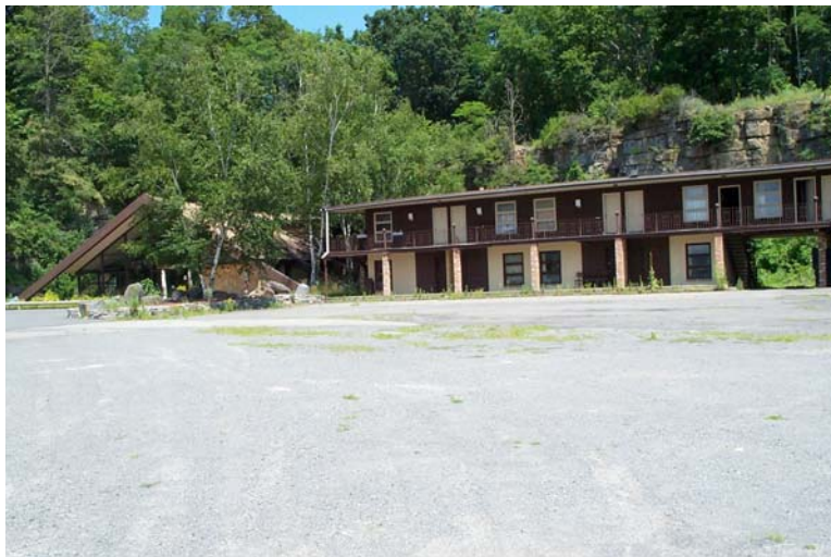
Motel units adjacent to restaurant/banquet facility that should have been demolished
