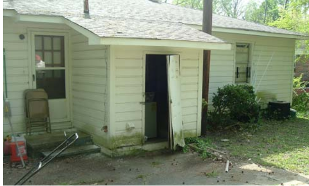
Damaged door on exterior laundry room used by the tenant poses a safety danger to the family and unauthorized access to the home.
