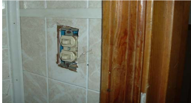
Light switch cover missing in the bathroom of unit where children live.
