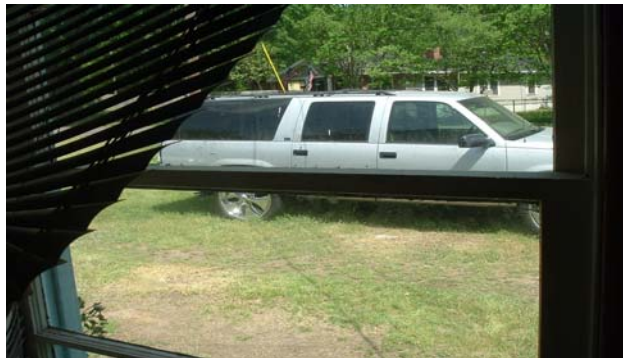
Window lock is missing.
