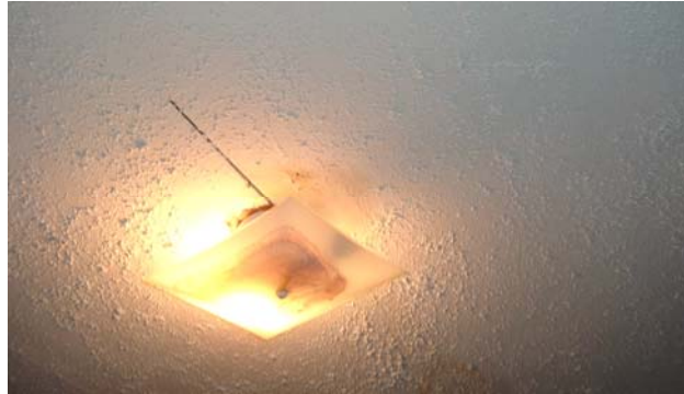
An active water leak from roof in light fixture with visible water damage to ceiling and fixture.
