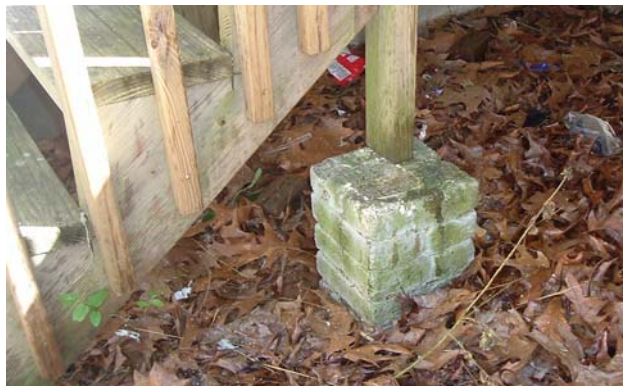
Stairs on deck not properly secured. The piling on the exterior deck was not set in concrete.
