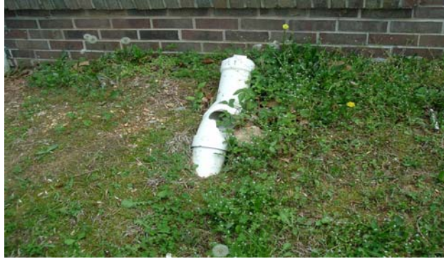
Broken and open sewer line on front of unit.
