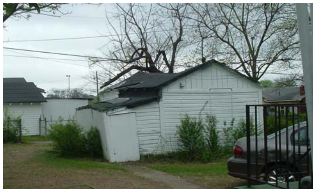
Roof collapsing on exterior storage building in the backyard where children play.
