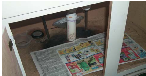
Pipe under sink actively leaking with visible mildew stains.
