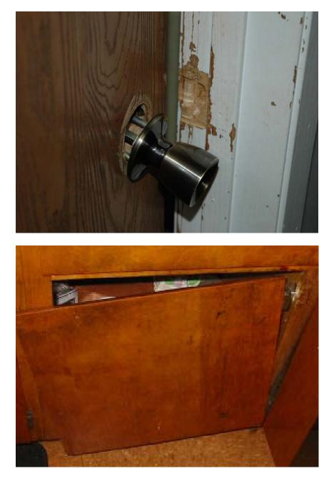
Unit #007-0722: cabinet door broken at hinge and will not close properly.
