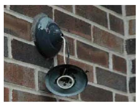
Unit #005-0437: missing outlet cover plate and outlet, exposing electrical contacts.
