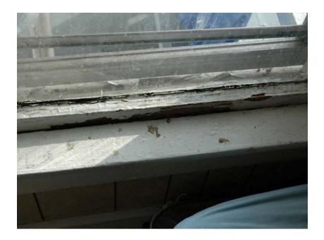
Unit #11: Loose spring track and cracked glass pane on the left front bedroom window.
