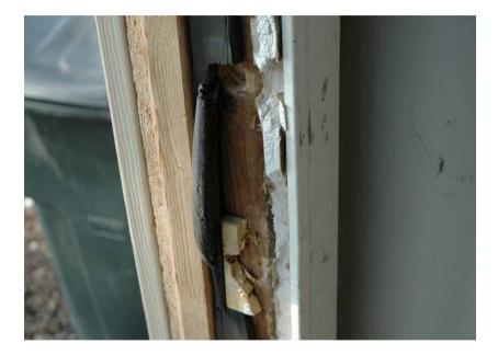
Unit #29: Missing latch bolt on door between kitchen and back porch.
