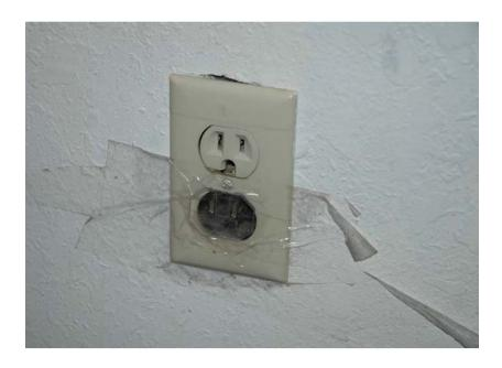
Unit #26: Broken outlet and improper wire connection to a rusted junction box without a cover plate.
