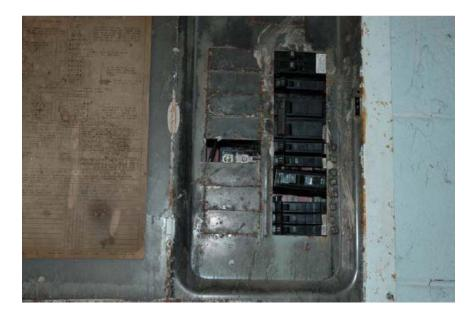
Unit # 5535: Unsecured cover on electric meter box and exposed electrical contacts.
