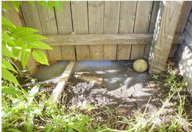
Unit occupied by the tenant and three children with raw sewage seeping from under the foundation.
