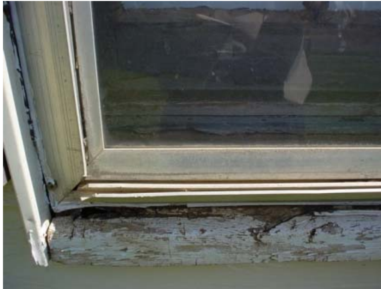
Unit in which the window sills on the entire house's exterior were deteriorated and dry rotted.
