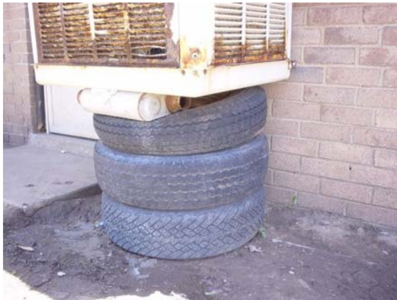
Unit in which the air conditioner was improperly supported.
