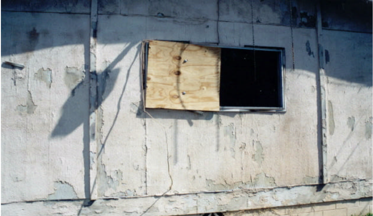
Photo 4: (046-674157) Exterior surfaces had extensive chipping and peeling paint. GFR's inspection reports did not identify any defective paint at the property.
