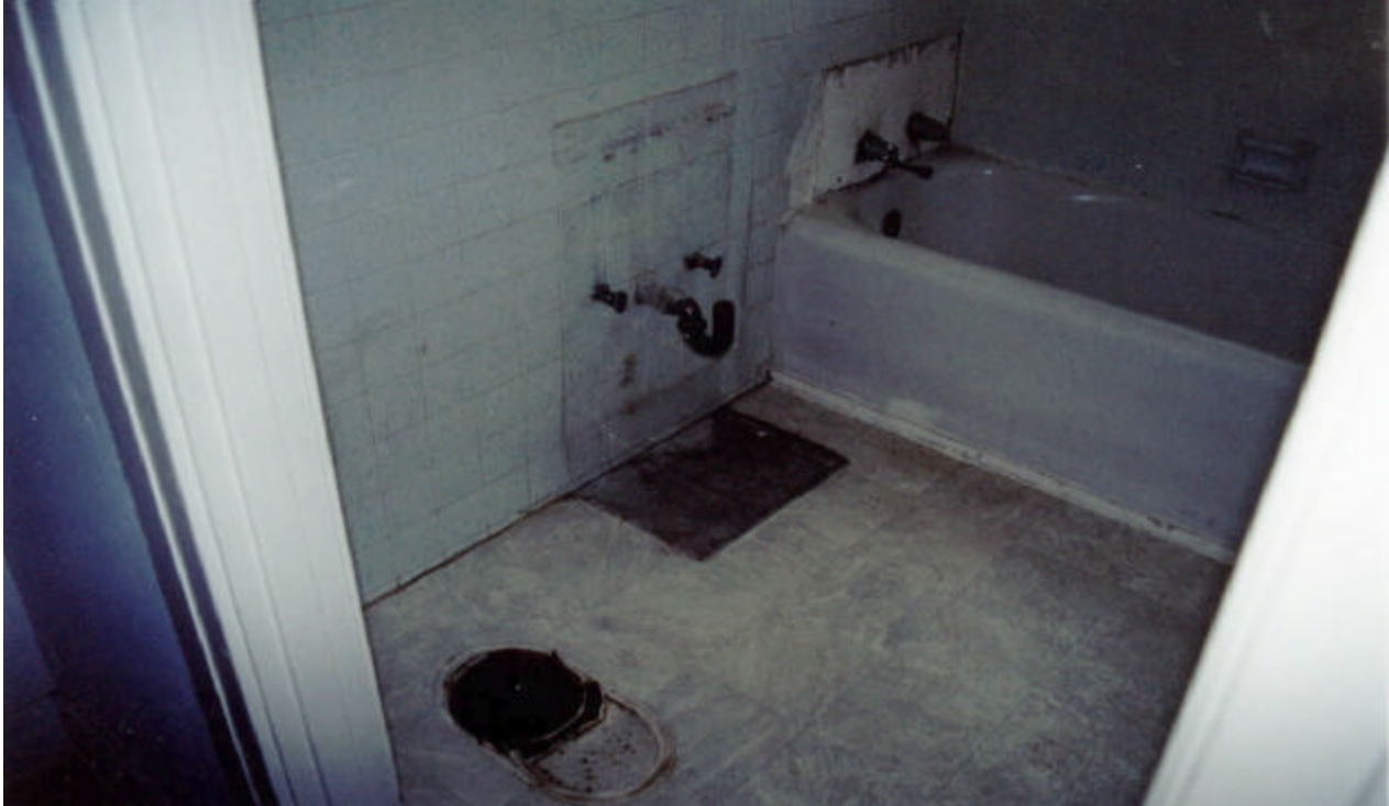
Photo 8: (197-041029) Property showed evidence of vandalism because of the missing bathroom sink, vanity, and toilet. GFR's inspection reports did not identify any missing items.
