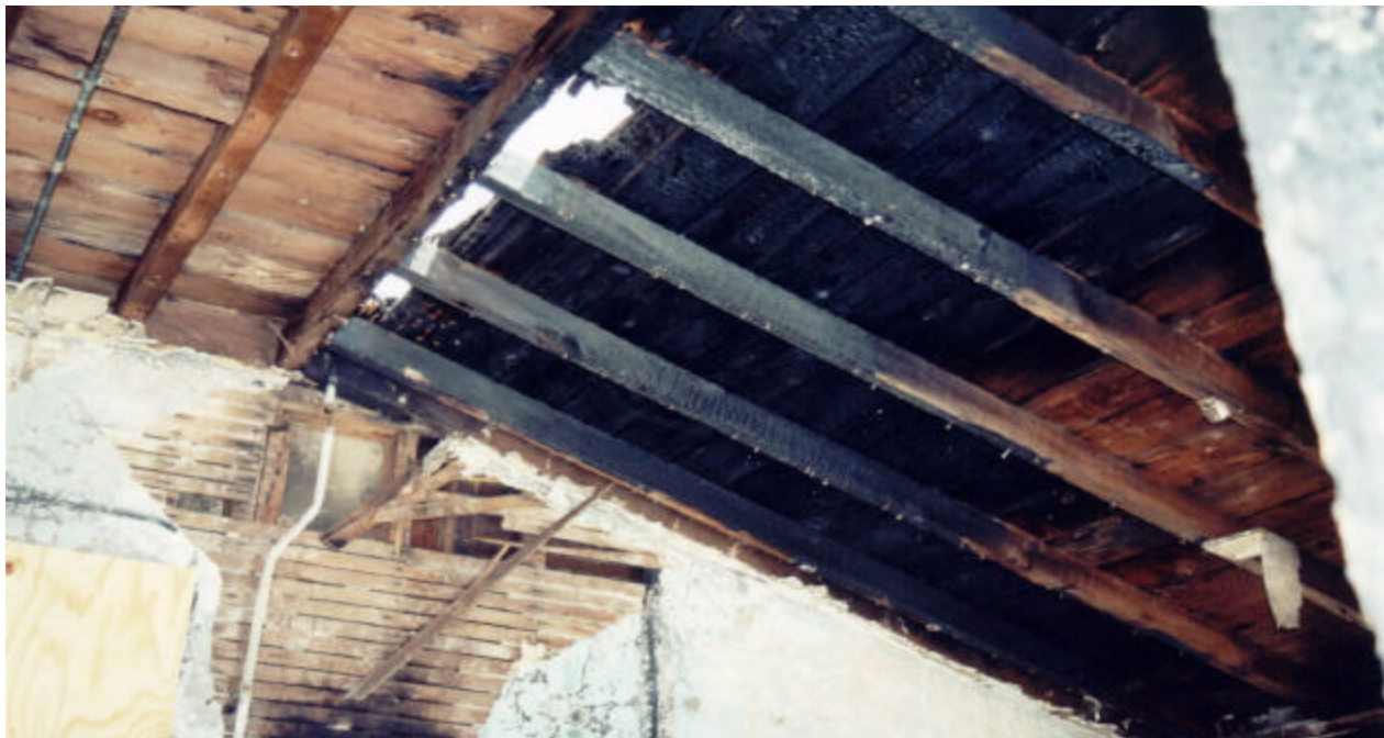
Photo 3: (041-963632) Rear stair case to the upper level unit is deteriorated and fire damaged, leaving it structurally unsafe. GFR's inspection reports did not report this deficiency.
