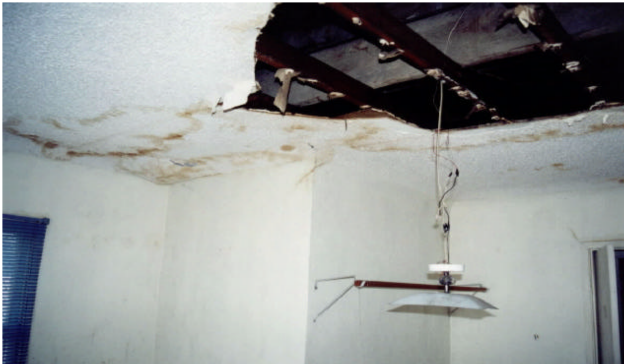
Photo 5: (041-984016) Property suffered extensive damage due to active roof leaks. GFR's inspection reports identified the need for repairs, but did not correct the problem.
