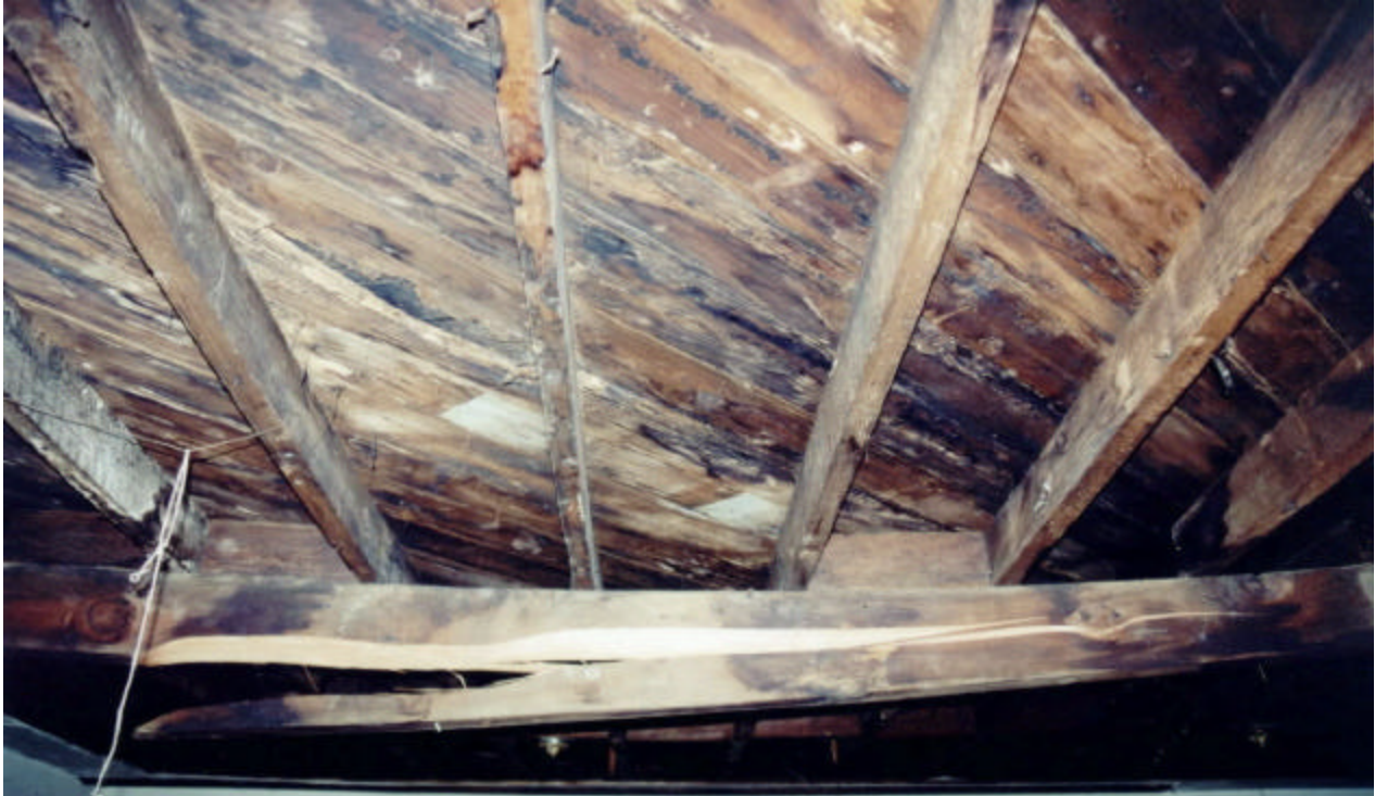
Photo 1: (041-941005) Garage support beam is severely split and very hazardous. GFR's inspection reports did not identify any safety hazards at the property.
