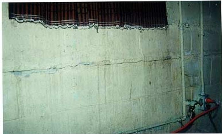
Foundation is severely cracked and a few inches out of alignment at 2126 Collingwood. This condition existed during the Housing Commission's last inspection.
