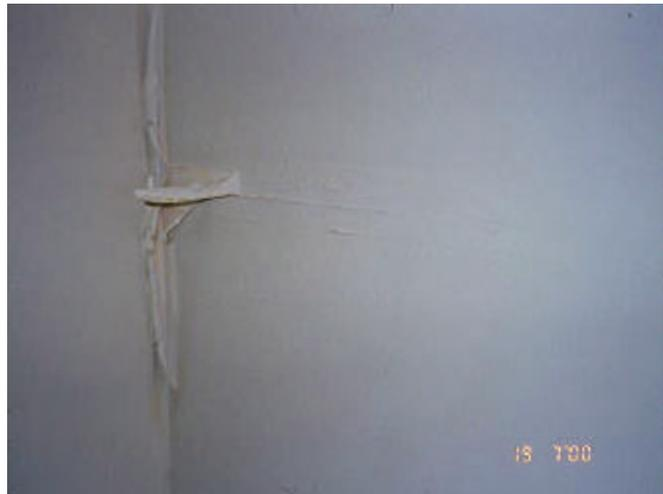
Water is leaking through the wall where the former steam pipes were located in the basement for Building 308.
