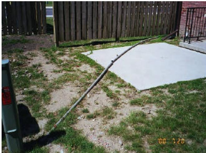
A rebar was extending up from the ground, which presented a hazardous condition near Building 501.
