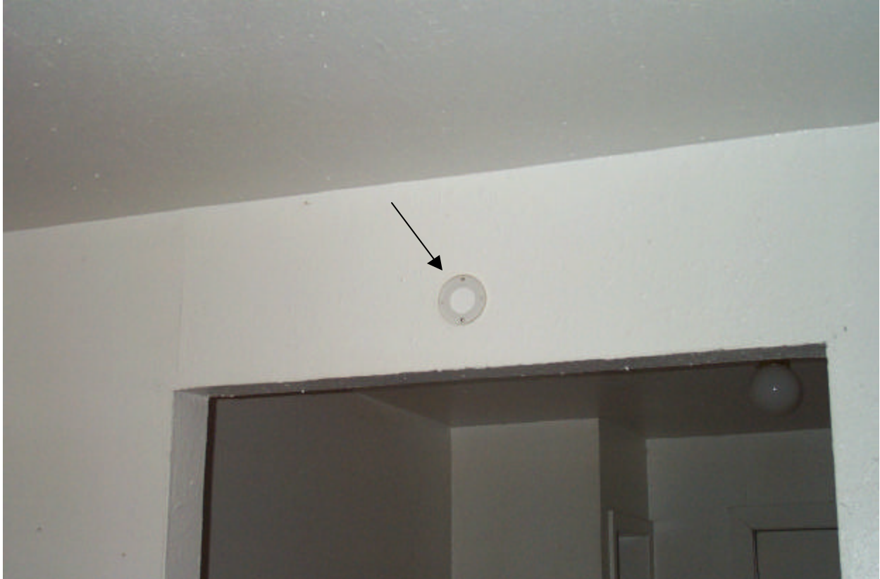
Figure 4: Unit 5712 - Missing smoke detector caused safety hazard
