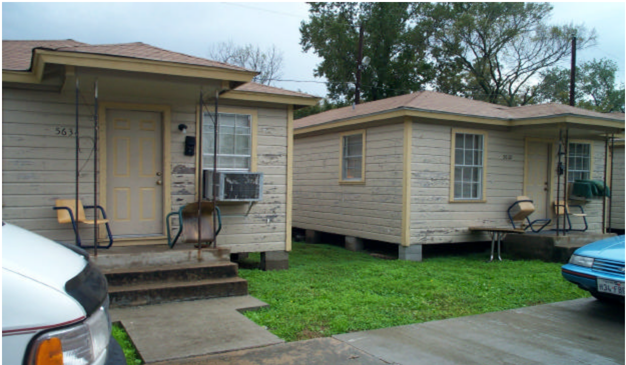
Figure 3: Outside Units - Cracked, peeling, deteriorated paint not decent or safe
