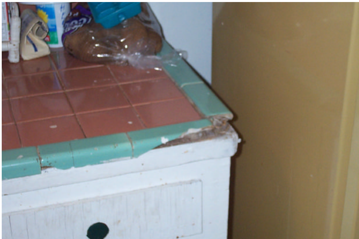
Figure 1: Unit 5704 – Chipped kitchen counter presented a safety hazard
