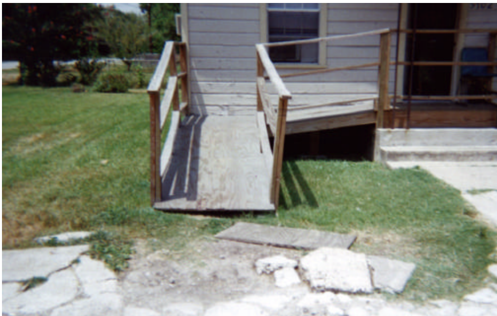
Figure 5: Office - Rocks and boards hindered access to handicapped ramps
