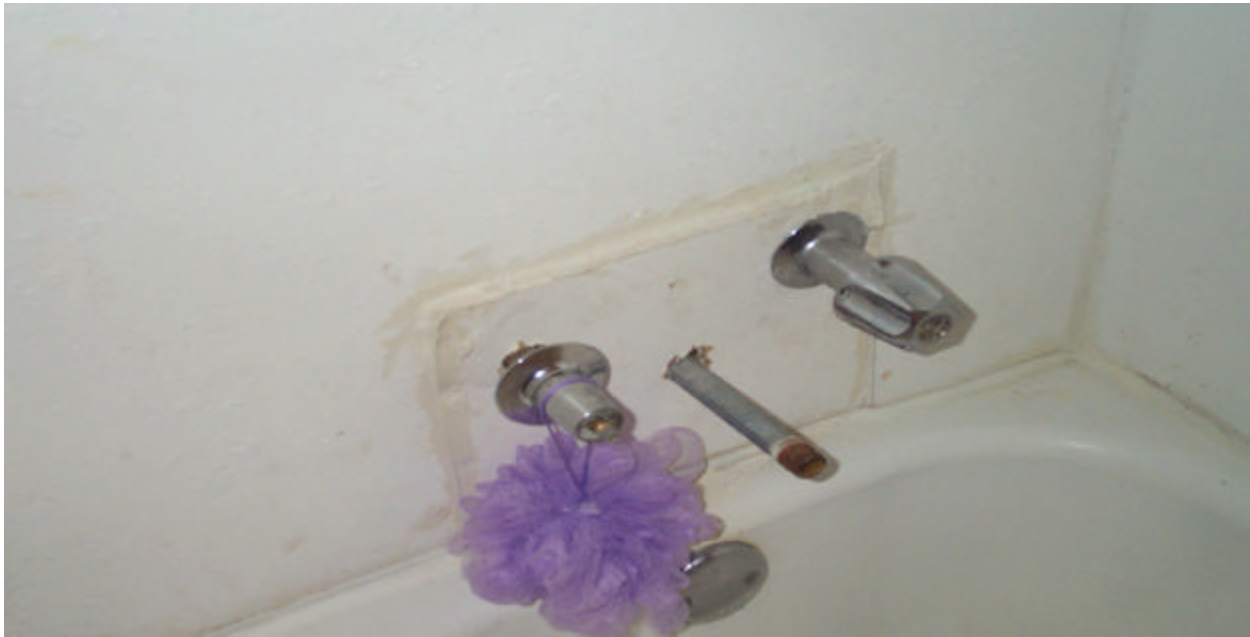
Figure 2: Unit 5712 - Missing handle and spout not sanitary
