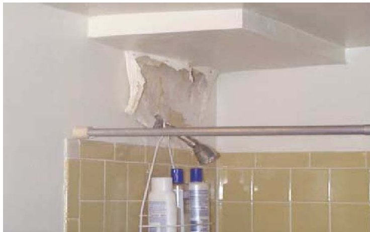
Paint peeling from the ceiling in one tenant's bathroom in Mitchell 66 Apartments.
