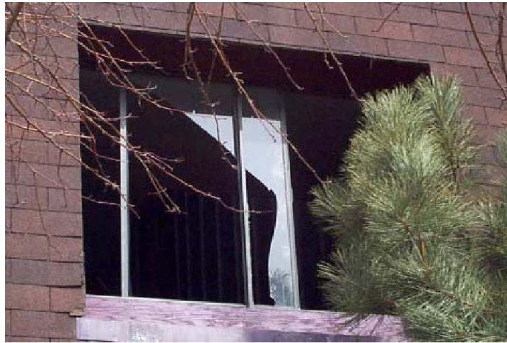
Broken window in a breezeway at Rotella Park Manor.
