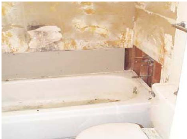
Tiles and bathtub parts taken from a vacant unit to replace parts in occupied units at Mitchell 66 Apartments.
