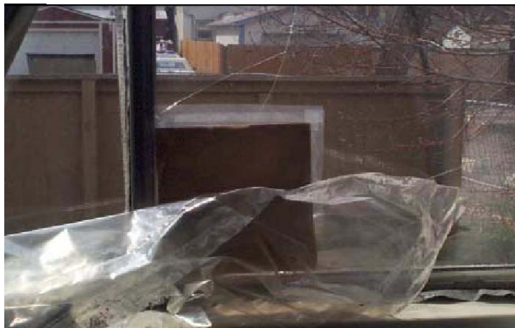
Broken window located in the infant's bedroom of an apartment at Denver Northeast Apartments.
