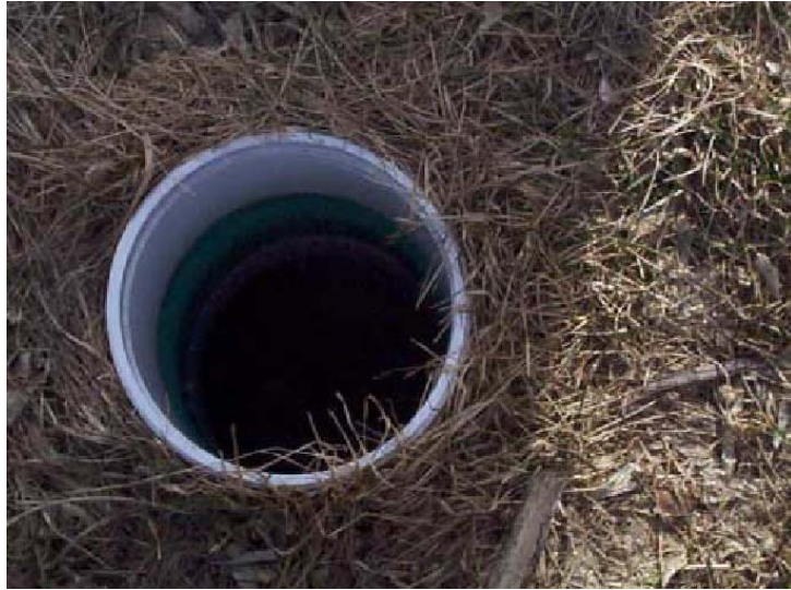
Uncovered drainage pipe located in front of one of the buildings at Rotella Park Manor.
