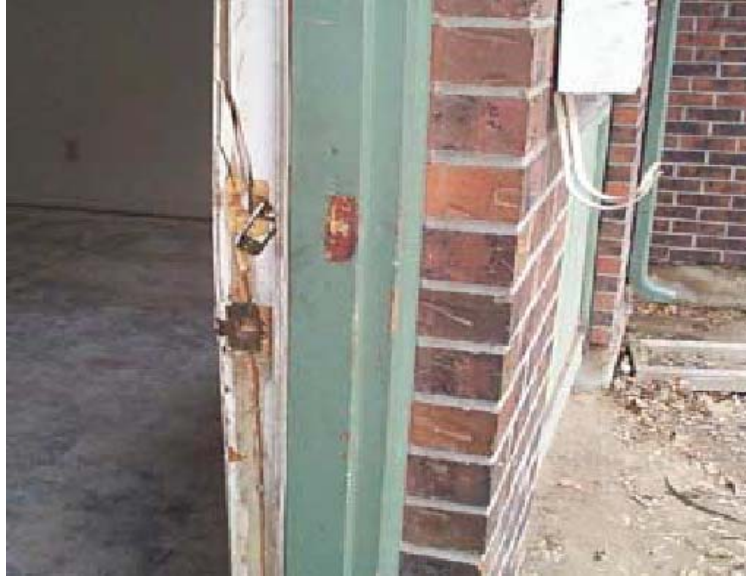
Damaged door jam of a vacant unit caused by someone kicking in the door.
