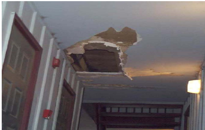
Water damage caused by broken boiler located in the hallway of a Rotella Park Manor building.
