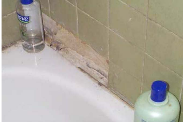
Tiles are missing from the bathtub of a unit in Mitchell 66 Apartments. Mold and mildew are in the grout areas of the bathtub.
