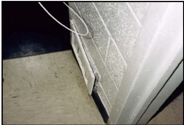
36 Lexington Drive (Lincoln Park) Loose vent in the rear bedroom
