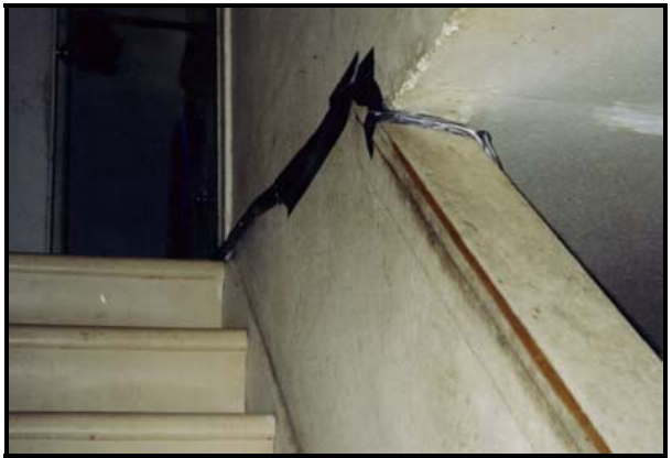
89 Swanson Drive (Swanson Homes) Phone cable on stairwell – tripping hazard
