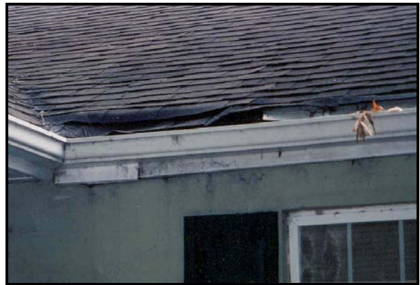
51 Dale Drive (after rehab) Roof sheathing damaged and leaking
