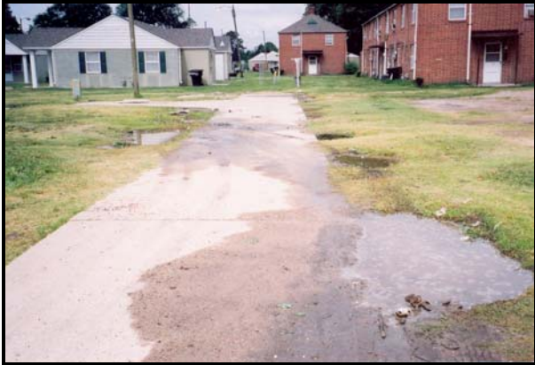
168 Dale Drive (after rehab) Ponding water and erosion from tire ruts in the common area sidewalks
