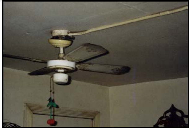
89 Swanson Drive (Swanson Homes) Broken ceiling fan in the living room
