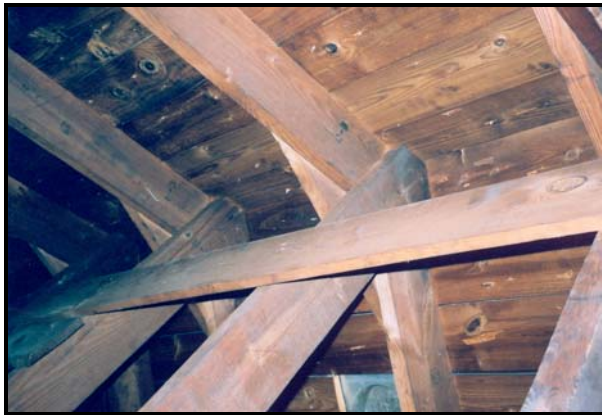
50 Dale Drive (after rehab) Roof without ridge vent and moisture stained decking
