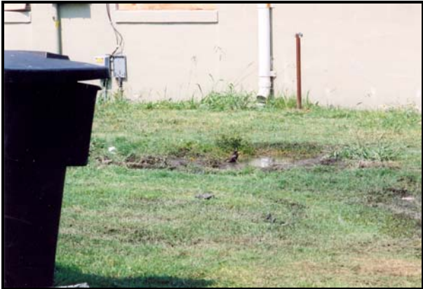
129 Dale Drive (after rehab) Standing water on site
