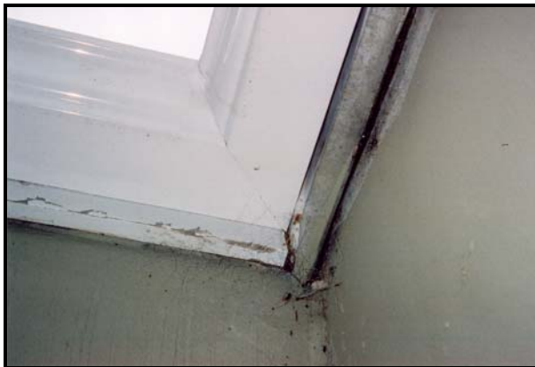
168 Dale Drive (after rehab) Water damage from gaps in fascia and drip edge at rear addition
