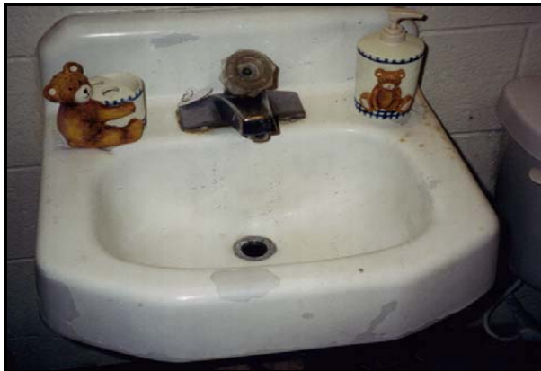
36 Lexington Drive (Lincoln Park) Peeling enamel on the sink in the first floor bathroom
