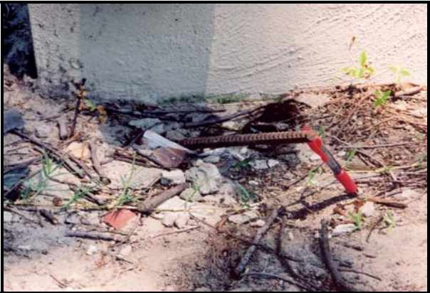
46 Dale Drive (after rehab) Rebar rods were exposed outside of the foundation and were a safety hazard
