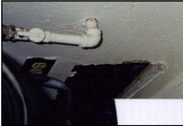
74 Merrimac (Swanson Homes) Pipe flange not sealed near the kitchen sink
