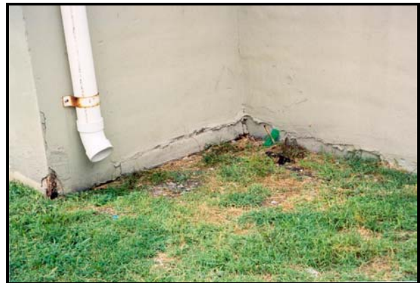
168 Dale Drive (after rehab) Exposed steel rebar missed the mark on the concrete pour Concrete parget chipping and cracking from corner and gaps left in stucco at foundation
