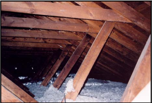
45 Dale Drive (after rehab) Area of roof sheathing in attic from previous water leak
