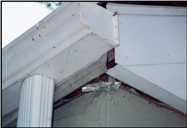
46 Dale Drive (after rehab) Exposed fascia left and no caulking was present
