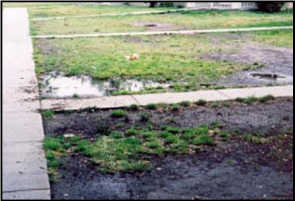
45 Dale Drive (after rehab) Standing water in common walkways area due to grading and traffic
