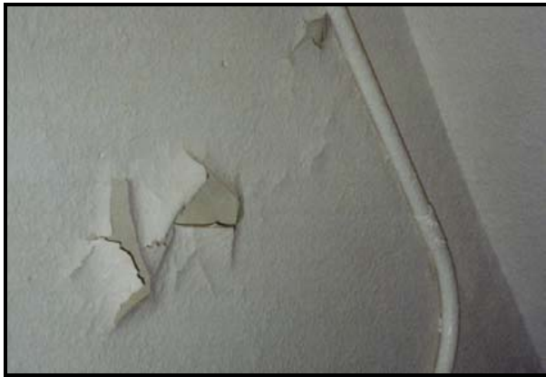
6 Merrimac Drive (Swanson Homes) Paint chipping on the bathroom ceiling
