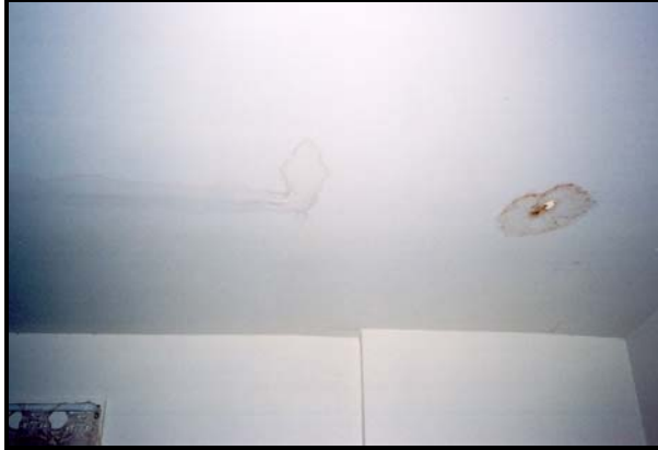
45 Dale Drive (after rehab) Stain from roof leak showing the kitchen ceiling damage
