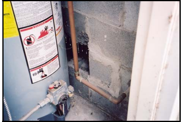
49 Dale Drive (after rehab) A concrete block was chipped and missing large pieces in mechanical room
