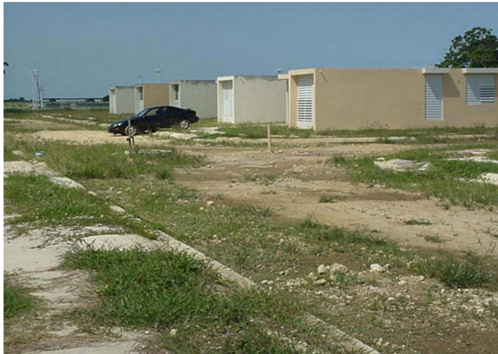
Partial view of houses under construction in block D.
