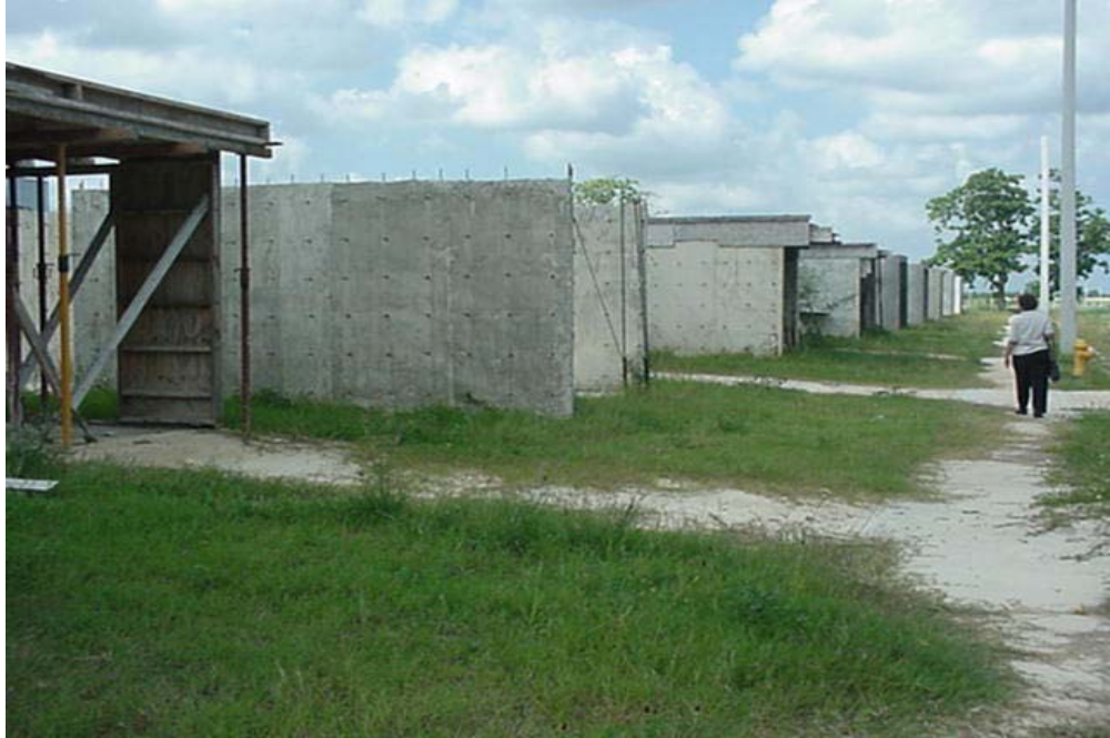
Partial view of houses under construction in block E.
