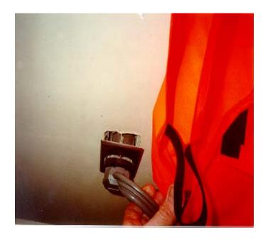
An electrical outlet had exposed wires because the cover plate was missing in the Public Housing unit located at 761 Magnolia Street.
