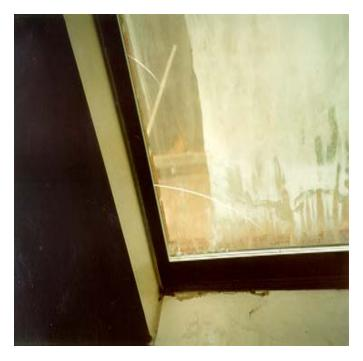
The Public Housing unit located at 911 Magnolia Street had a missing window seal which allowed air infiltration into the unit.
