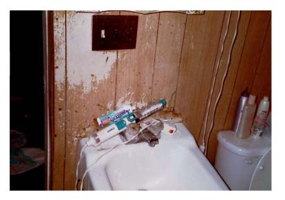
No GFCI outlet installed in the bathroom at 235 West 4<sup>th</sup> Street.
