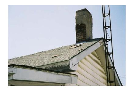
Roof fascia and brick chimney had excessive wear and were in need of repair at 321 Grand Avenue.
