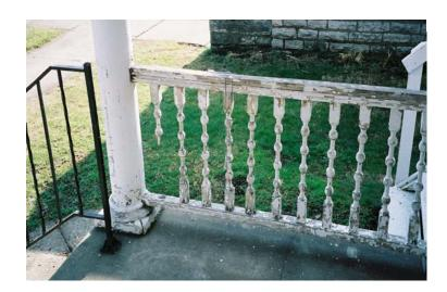
The porch railings and posts were broken, rotted, and deteriorated at 207 West 4<sup>th</sup> Street.
