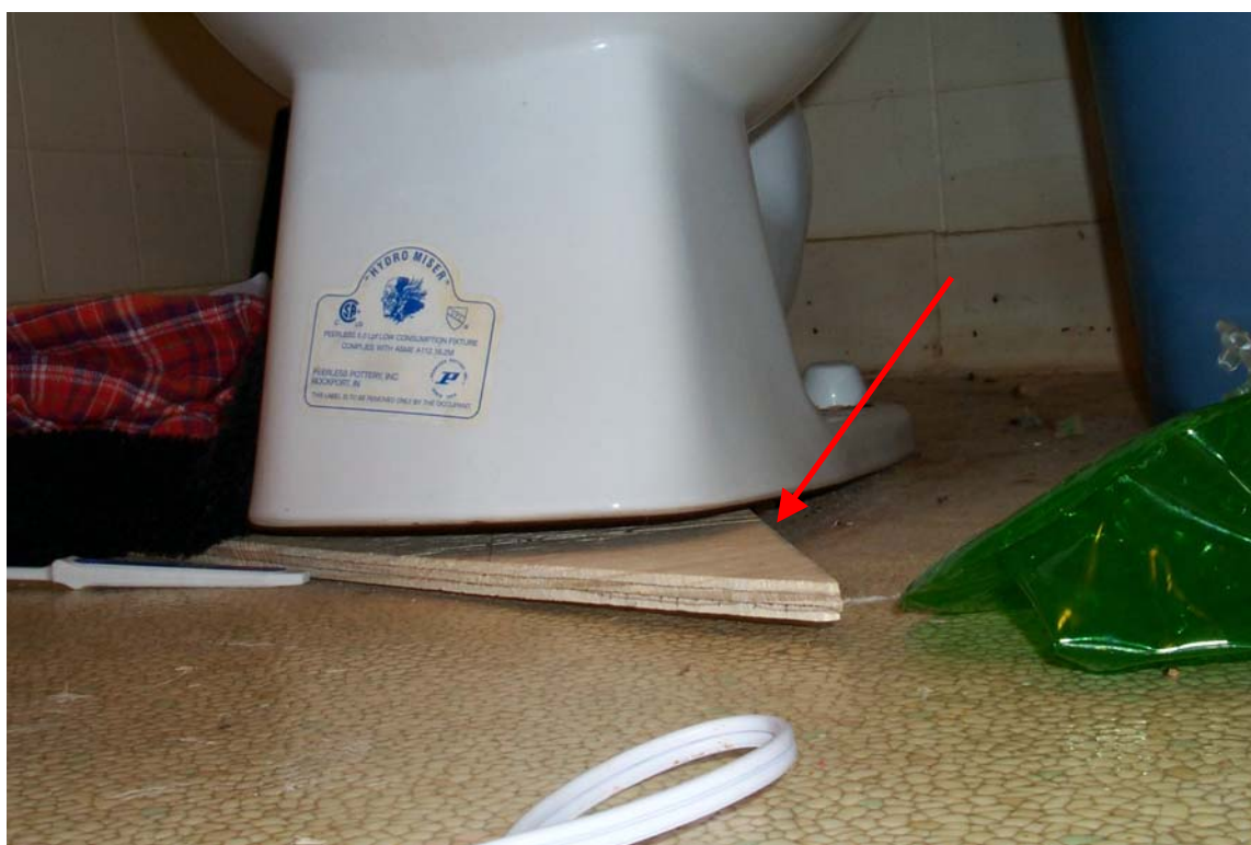
Photo 11 The toilet was not professionally installed. It is stabilized with plywood to prevent rocking. Contractor received $3,375 to upgrade the plumbing and replace fixtures.
