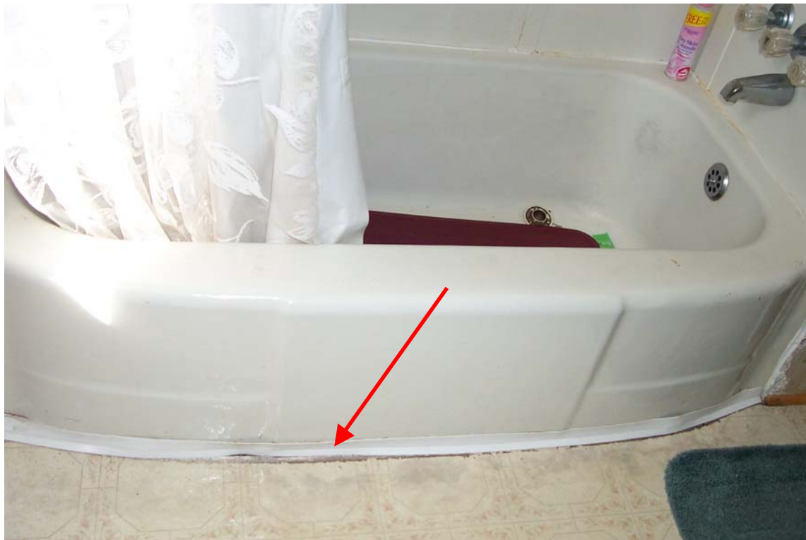
Photo 13 Contractor installed white, rubber weather-stripping to cover the gap between the bathtub and the floor. Contractor received $3,375 to upgrade the plumbing and replace fixtures.
