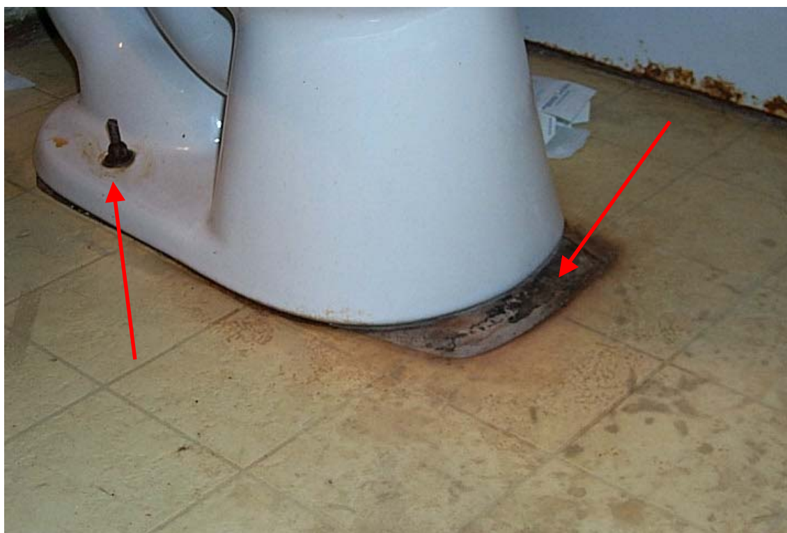
Photo 6 Contractor unprofessionally installed the toilet. Contractor received $3,675 to upgrade plumbing and install new fixtures.
