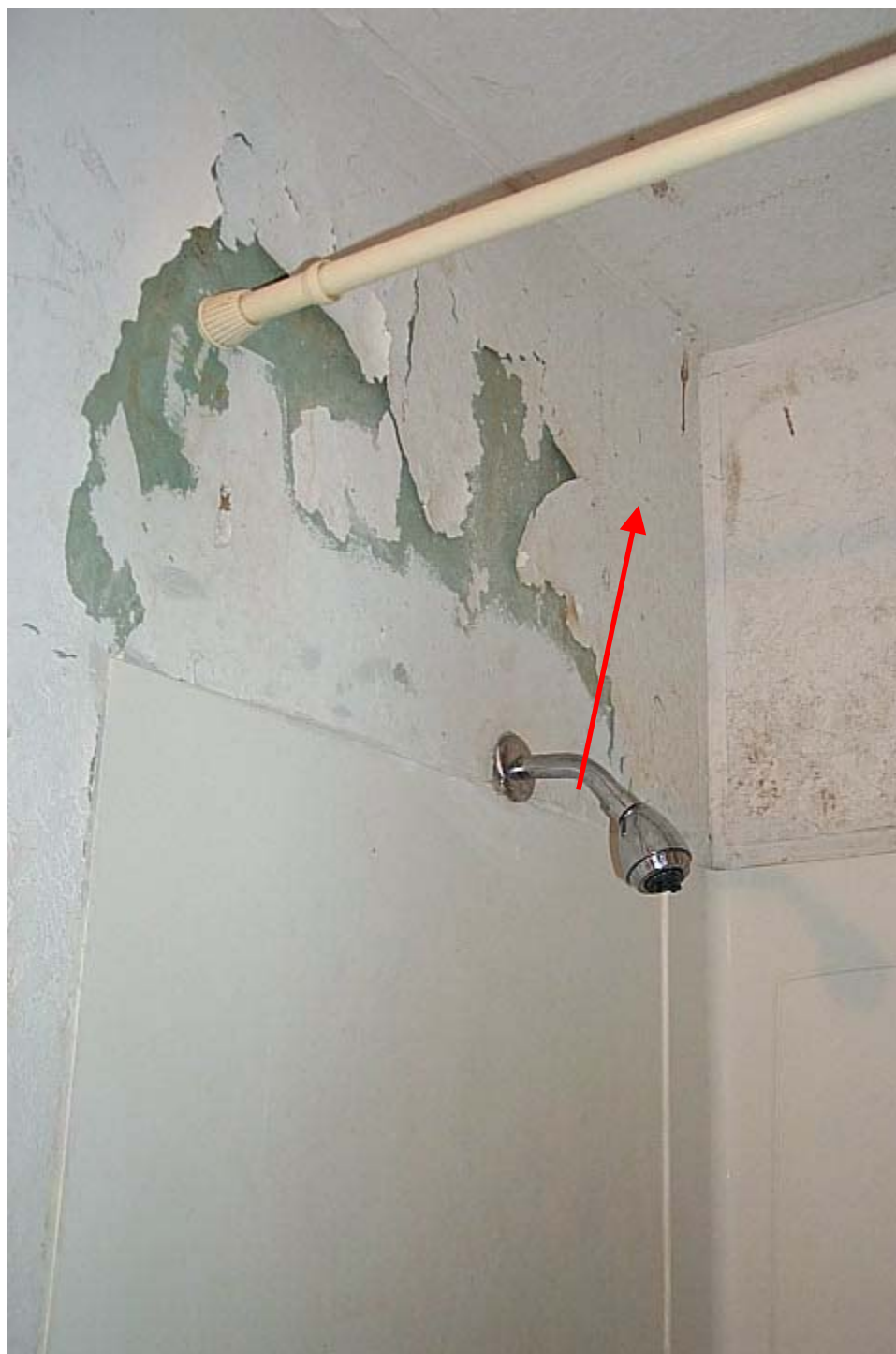
Photo 9 Homeowner's wall is deteriorating. Contractors did not fix this problem. Contractors billed a total of $5,266 to rehab the home.
