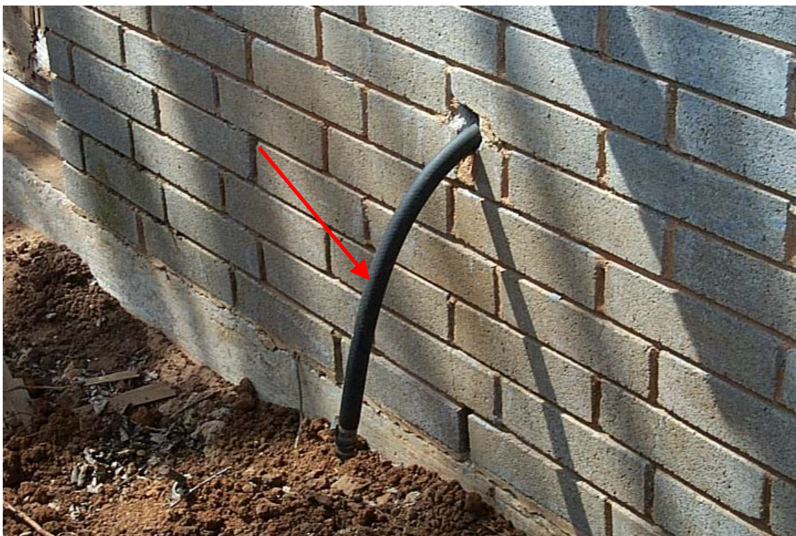
Photo 8 Contractor did not fix the makeshift dishwasher drain. Contractor received $3,375 to upgrade the plumbing.
