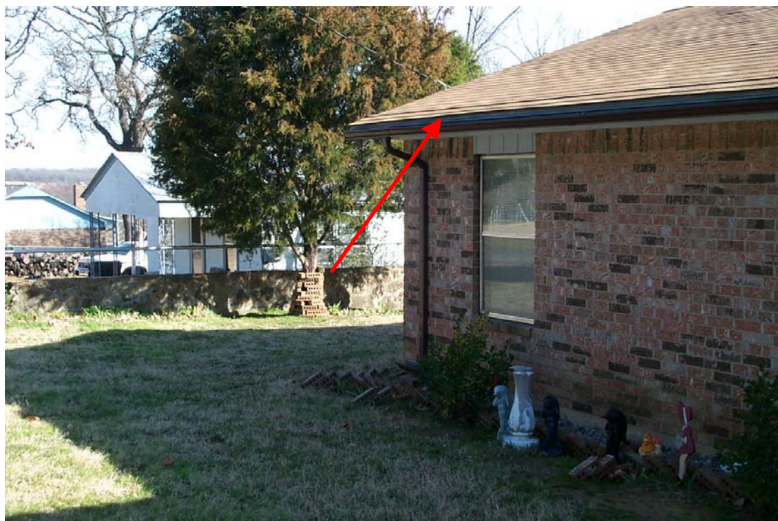
Photo 15 Contractor received $721.50 to install gutters although original gutters were not replaced.
