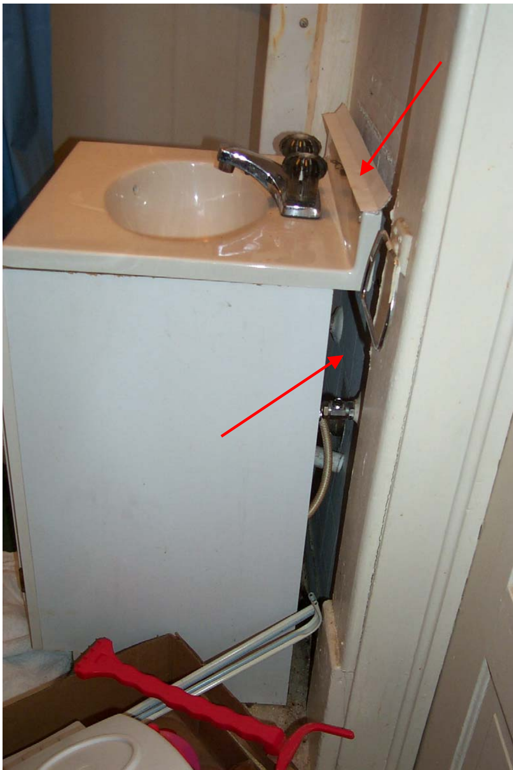
Photo 12 Sink and cupboard are not professionally installed. There is a large gap behind the sink and cupboard. Contractor installed white, rubber weather-stripping to cover the gap between the top of the sink and the wall. Contractor received $3,375 to upgrade the plumbing and replace fixtures.
