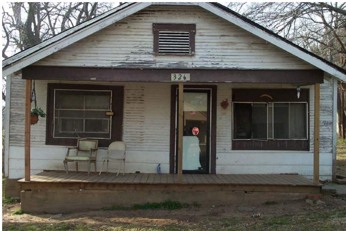
Photo 3 Contractor received $850 to bring attic insulation up to code although insulation is still missing 8-inches. Contractors billed a total of $8,630 to rehab the home.
