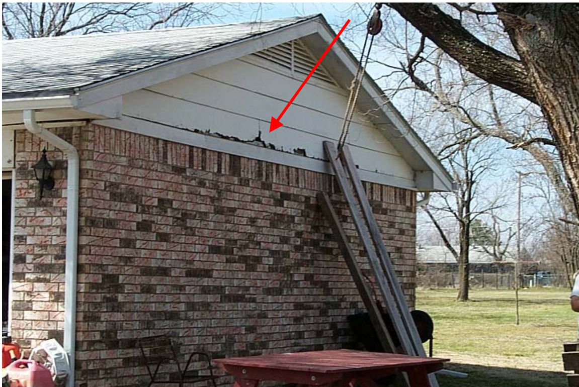
Photo 7 Birds continue to nest inside the home. Contractors billed a total of $9,925 to rehab the home.
