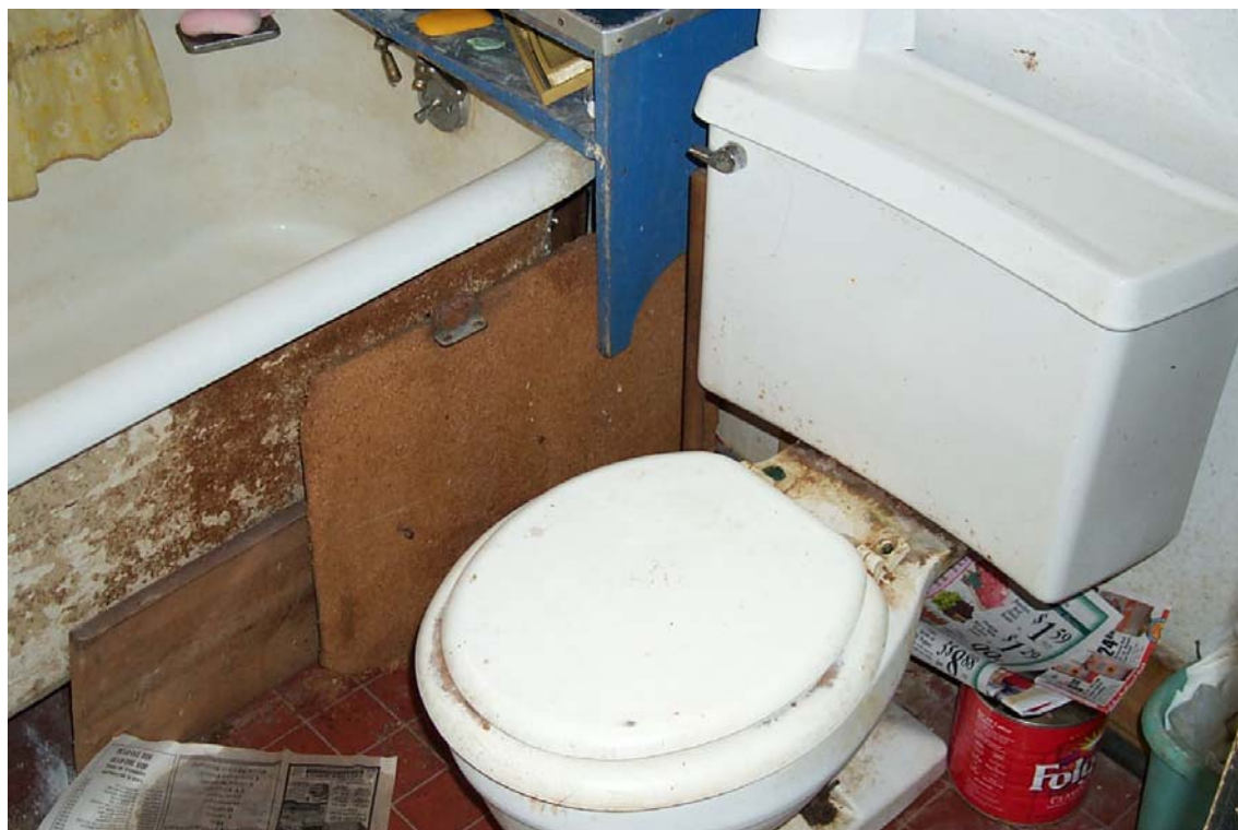
Photo 4 Contractor received $3,875 to upgrade the plumbing although no plumbing work was performed.
