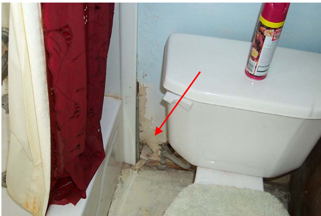
Photo 5 Homeowner's wall is deteriorating. Contractors did not fix this problem. Contractors billed a total of $7,999 to rehab the home.
