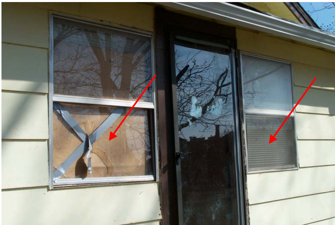
Photo 10 Contractor received $4,725 to replace 15 windows. These two windows were not replaced.
