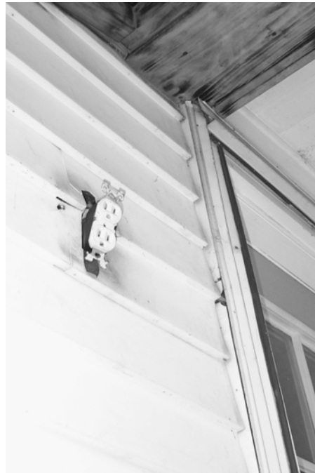
Exterior Outlet Non GFI – 43 Talcott Avenue
