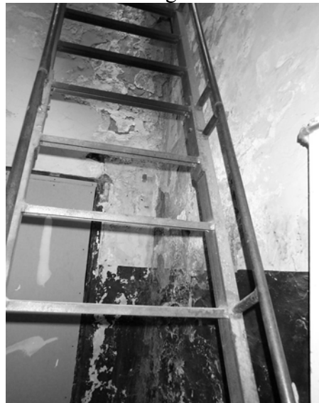
Excessive Peeling Paint in Hallway – 140 Chestnut St.
