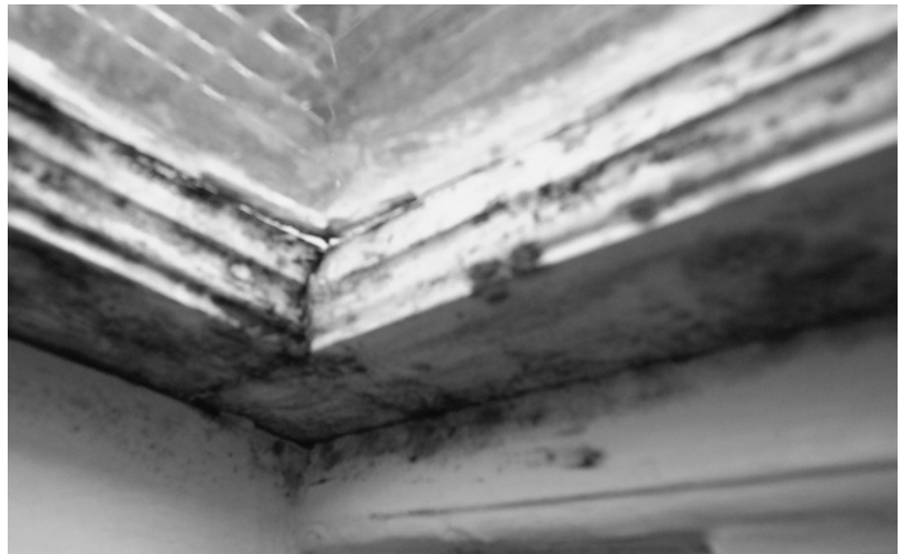
Mold underneath side window - 26 Ambrose Street
