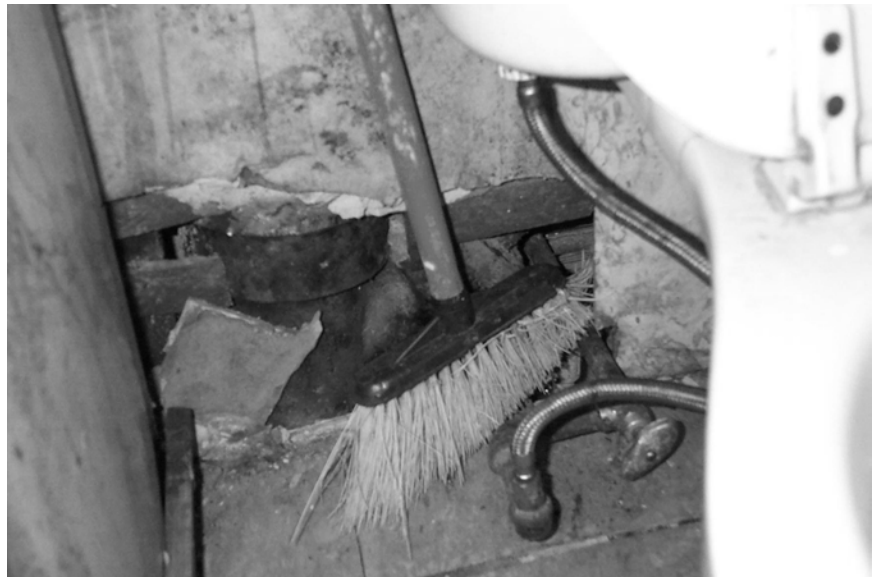
Hole in Bathroom Floor - 18 Phoenix Street
