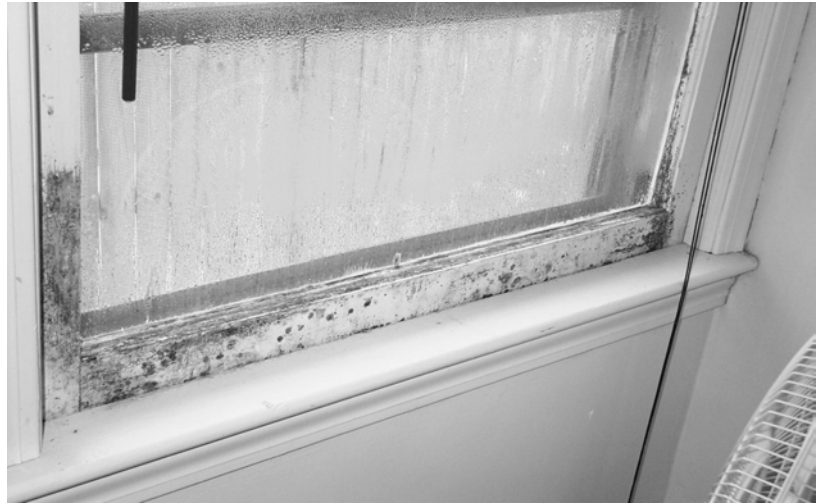
Mold on windows - 26 Ambrose Street
