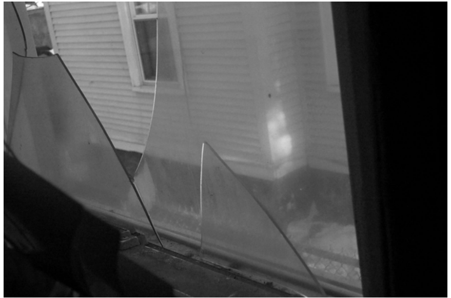
Broken Window - 18 Phoenix Street
